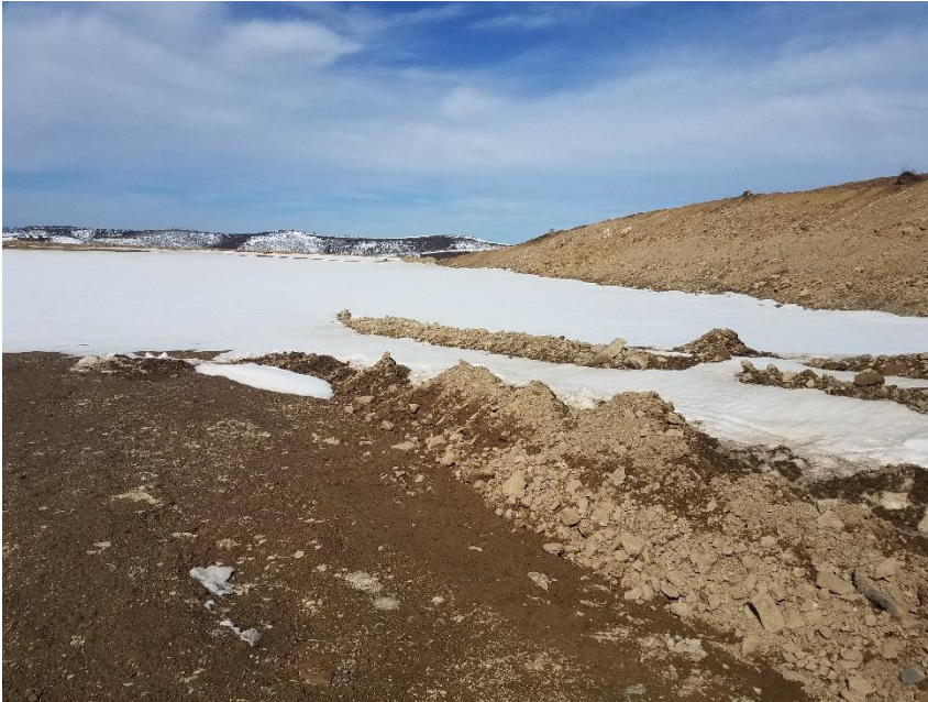
Photo 3: See comments under photo 1. Photo also shows topsoil stockpile on the north end of the Location; No stormwater or stabilization controls have been installed on the soil stockpiles in accordance with Rule 1002.f
