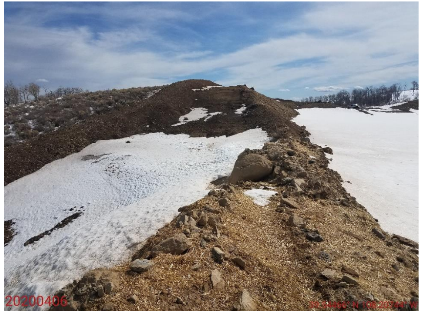
Photo 6: Photo taken from the northwest end of the Location, facing east. Photo shows topsoil stockpile on the north end of the Location; No stormwater or stabilization controls have been installed to protect the soil stockpiles in accordance with Rule 1002.f
