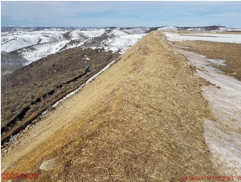
Photo 5: Photo taken from the south end of the Location, facing west. Photo shows straw mulch has been installed to stabilize and protect the fill slopes of the Location.
