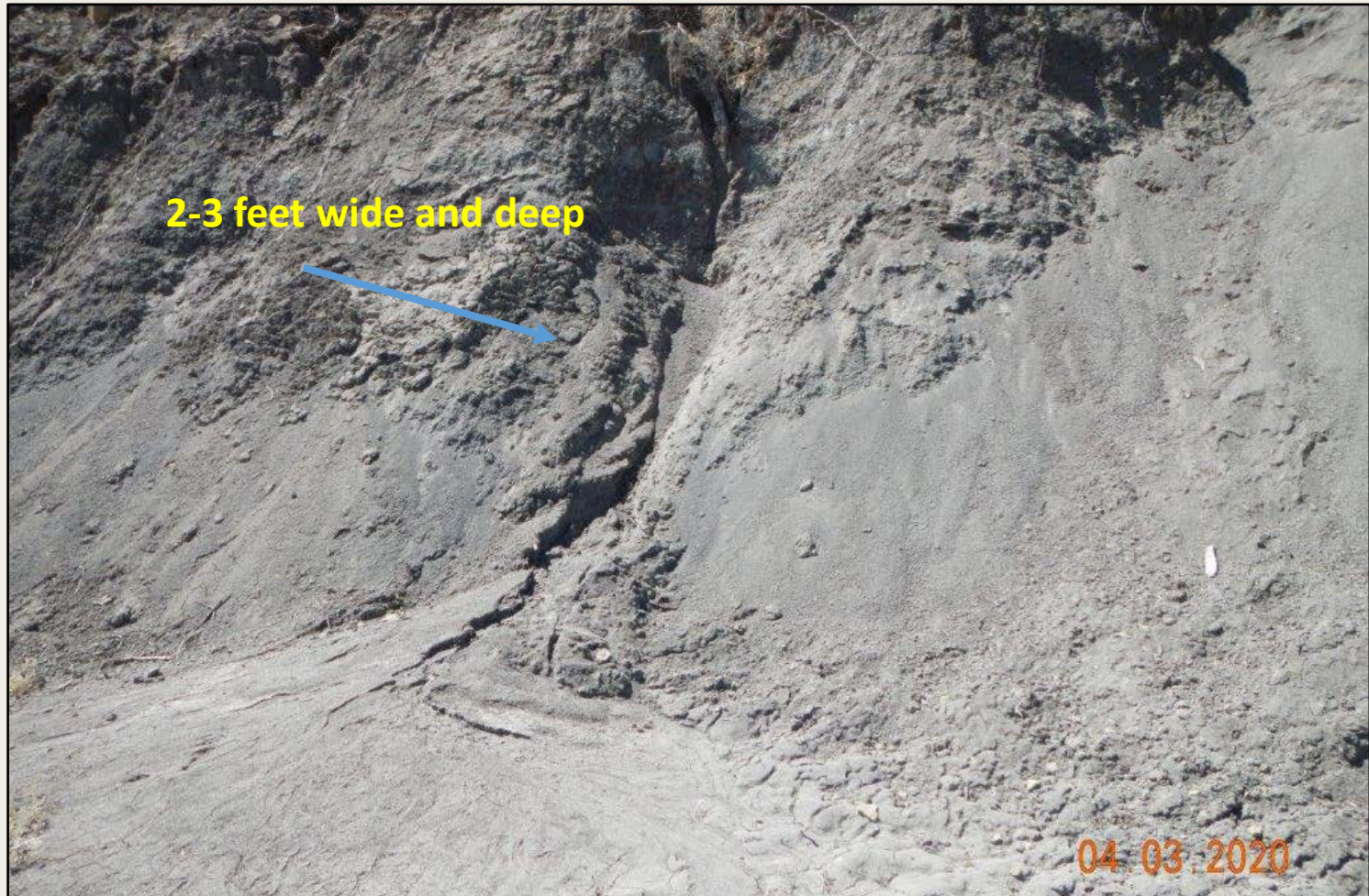
Photo 3. View of erosion and sediment deposition on western cut-slope.
