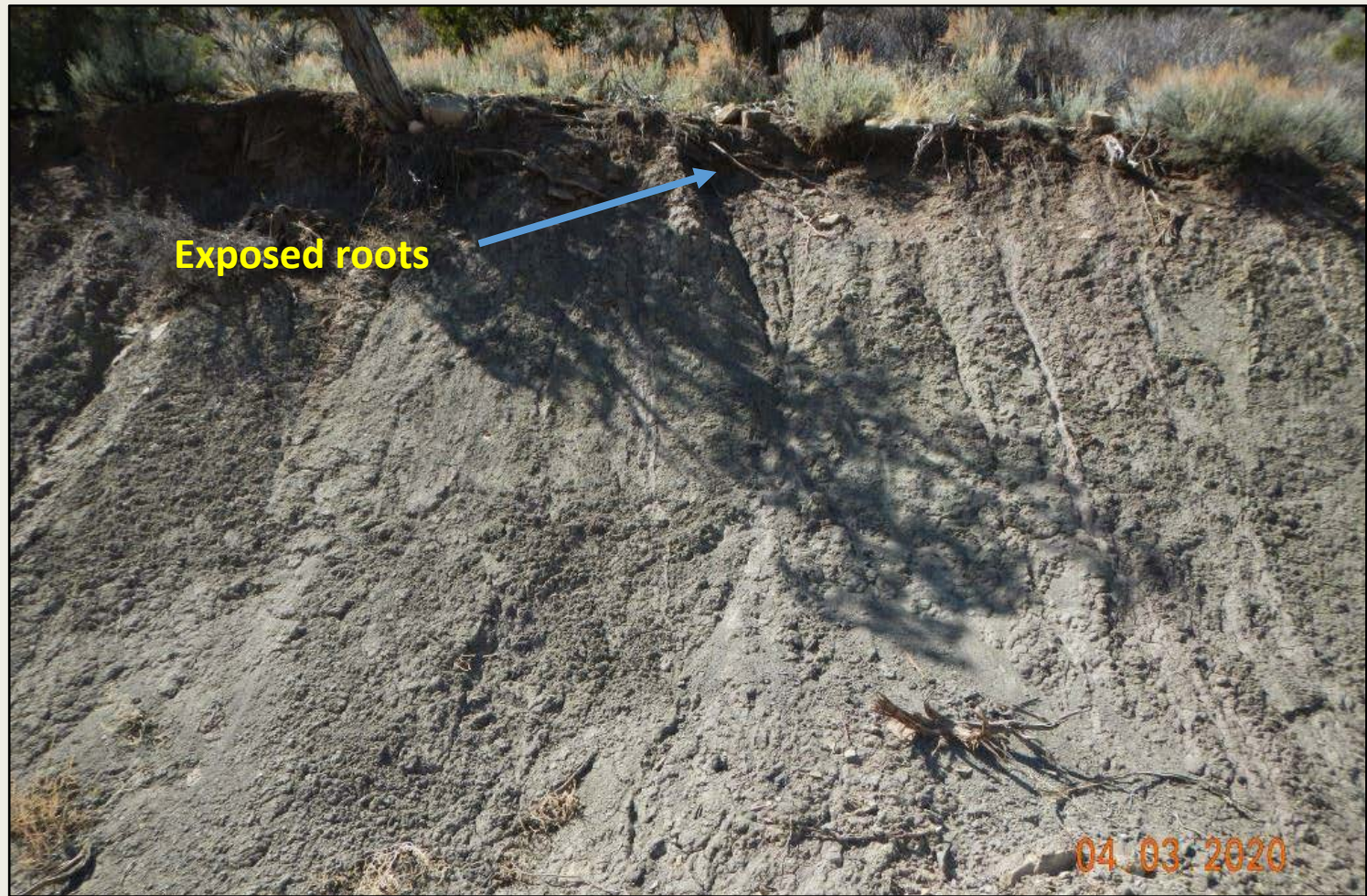
Photo 5. View of bare soils and exposed roots on cut-slope.
