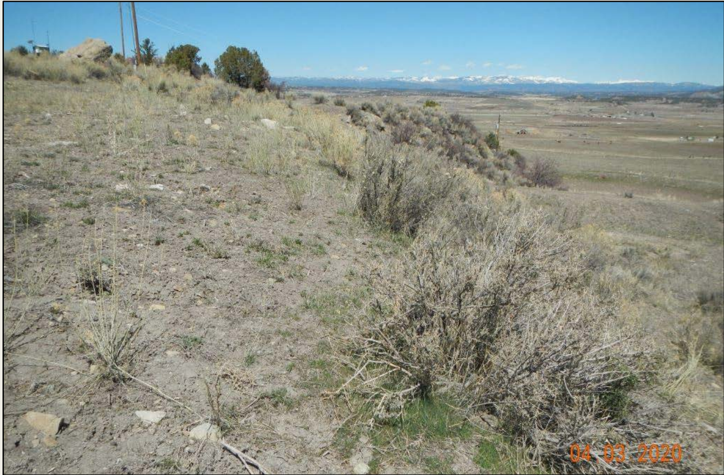
Photo 9. View of the eastern fill slope, facing northward. Revegetation is comprised of shrubs such as rubber rabbitbrush, as well as cheatgrass, and other perennial grasses such as crested wheatgrass.
