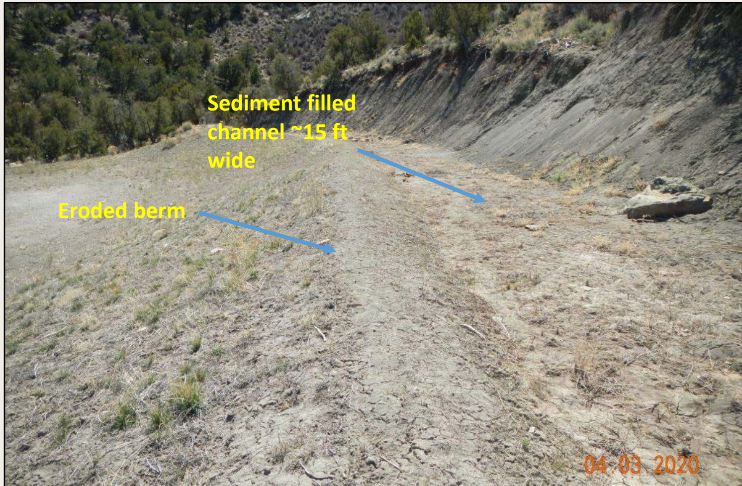
Photo 2. View of the western cut-slope and diversion channel. Slope and berm eroding and channel is full of sediment.
