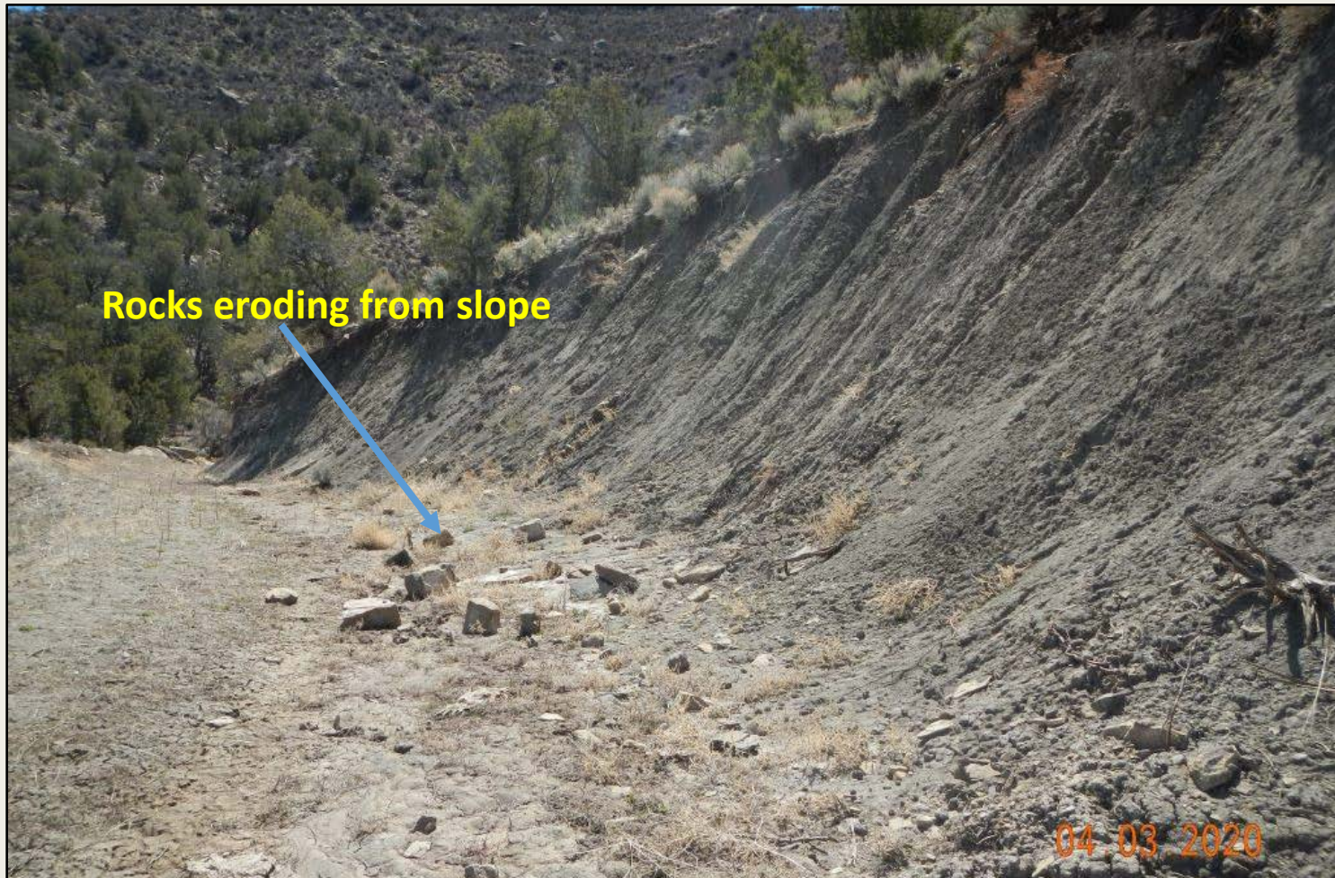
Photo 4. Another view of well pad cut-slope and sediment-filled diversion. Rocks at toe of slope appear to be eroding from slope above.
