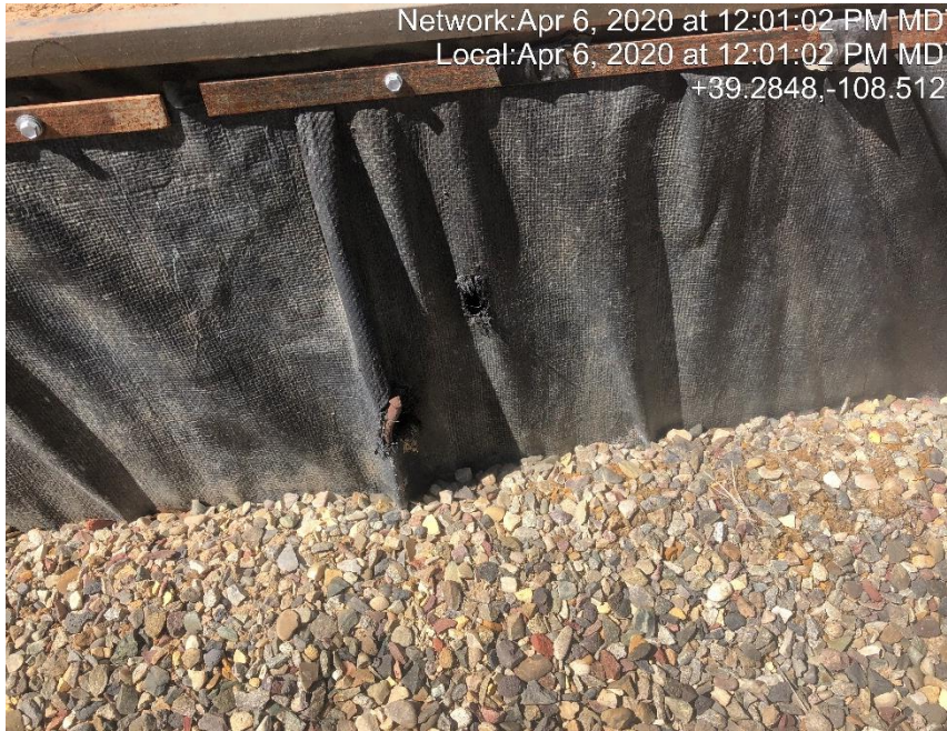
Photo #0905 Holes in tank containment liner.
