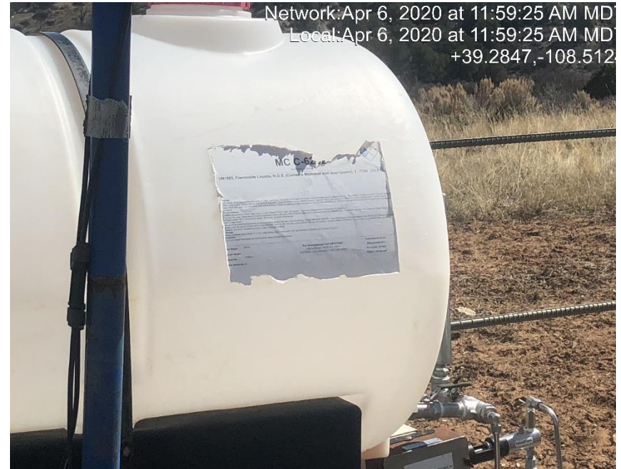
Photo #0904 Chemical tank NFPA label weathered and not legible.
