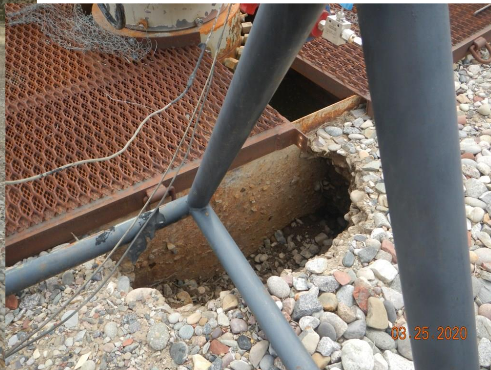
Photo#4: Subsidence at Well API#045-22157.
