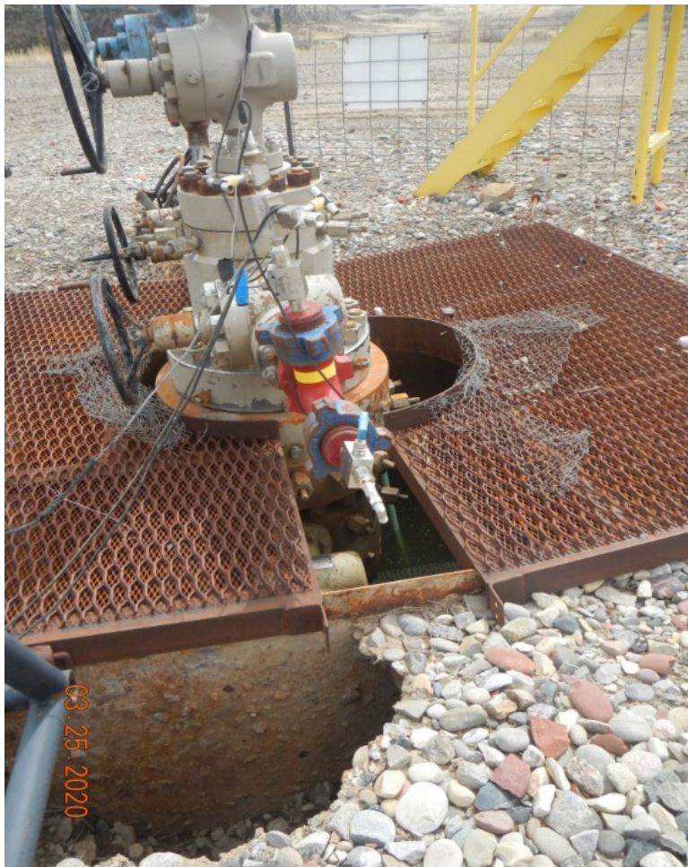
Photo#5: Cellar grates (covers) are not complete.
