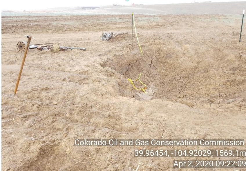
Photo 7 Open excavation around well head no safety fence of storm water BMP's in place.
