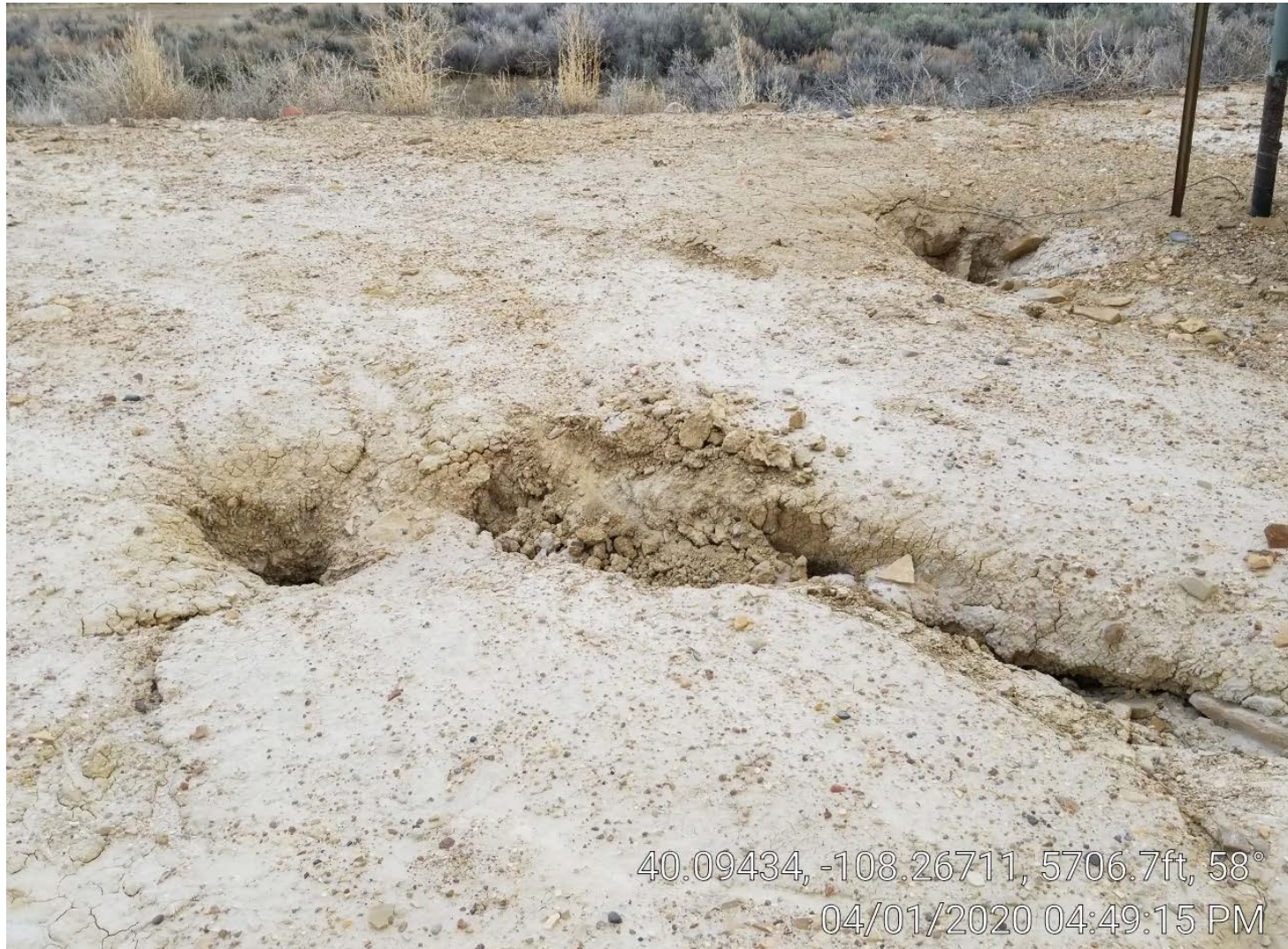
Photo 4. Storm water channel s & holes by meter building.
