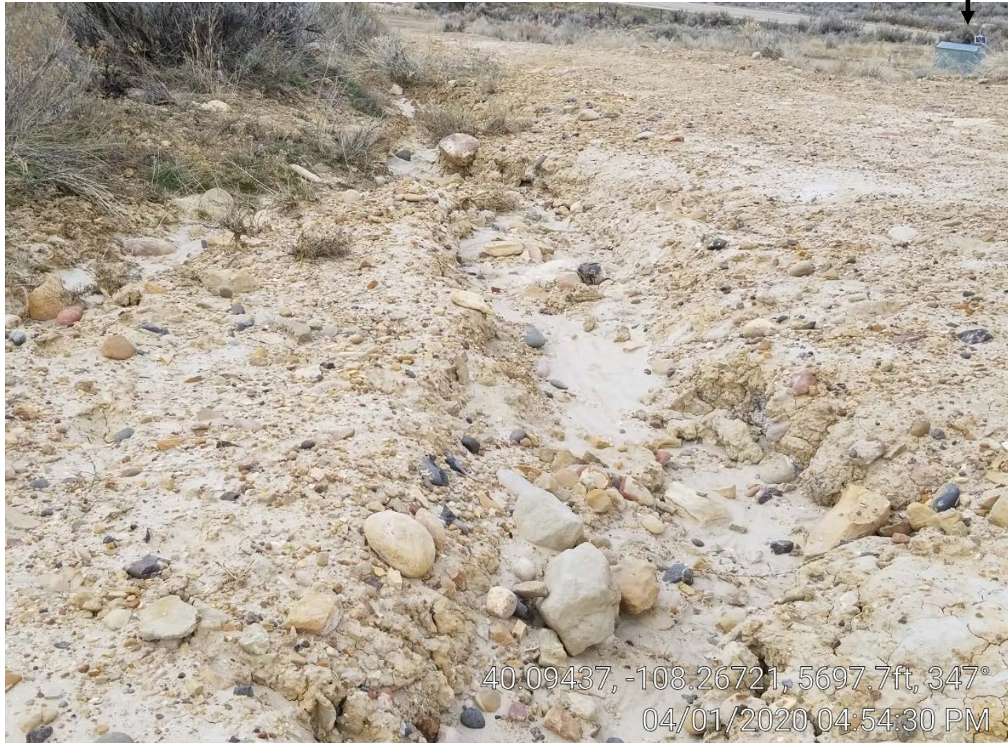
Photo 5. Storm water channel coming off location down access road.
