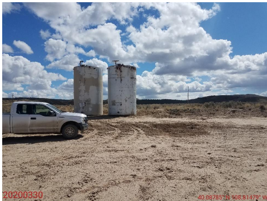
Photo 1: Photo taken from the east end of the Location, facing south. Photos 1-4 provide an overview of the Location from south, southwest, northwest to north. Location appears to have been PA in 2018. Photo shows equipment remaining on the Location and no reclamation activities appear to have been conducted in accordance with COGCC 1004 rules.
