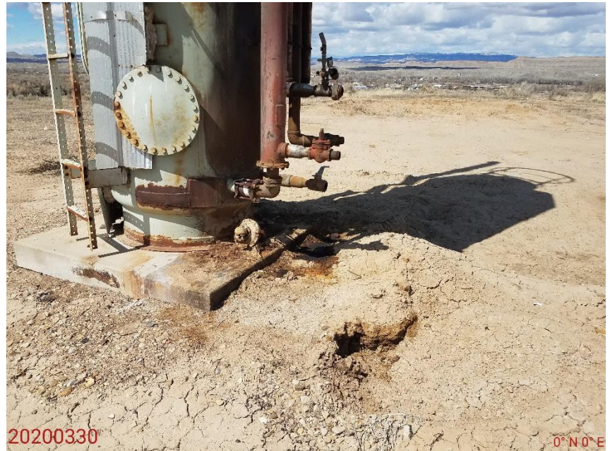
Photo 10: Continued from photo 9. Photo shows stained soils due to leaks from unused equipment.
