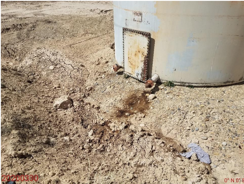
Photo 13: Photo shows stained soils due to leak from tanks.
