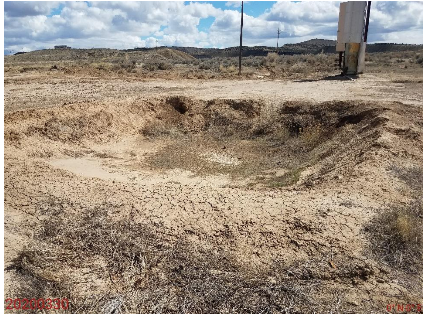
Photo 8: Photo taken from the west end of the Location, facing south. Photo shows a pit remains open on the Location.
