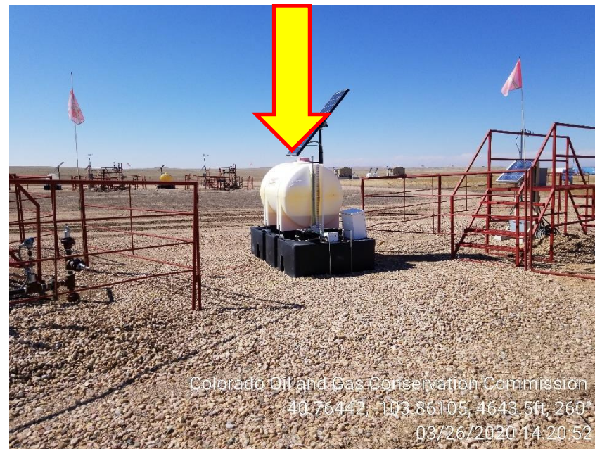
Photo 4 – Eastside Chemical tank – missing/faded Label
