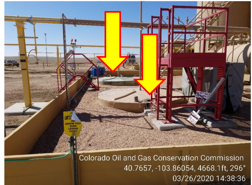
Photo 10 – Produced Water Tanks missing Signage
