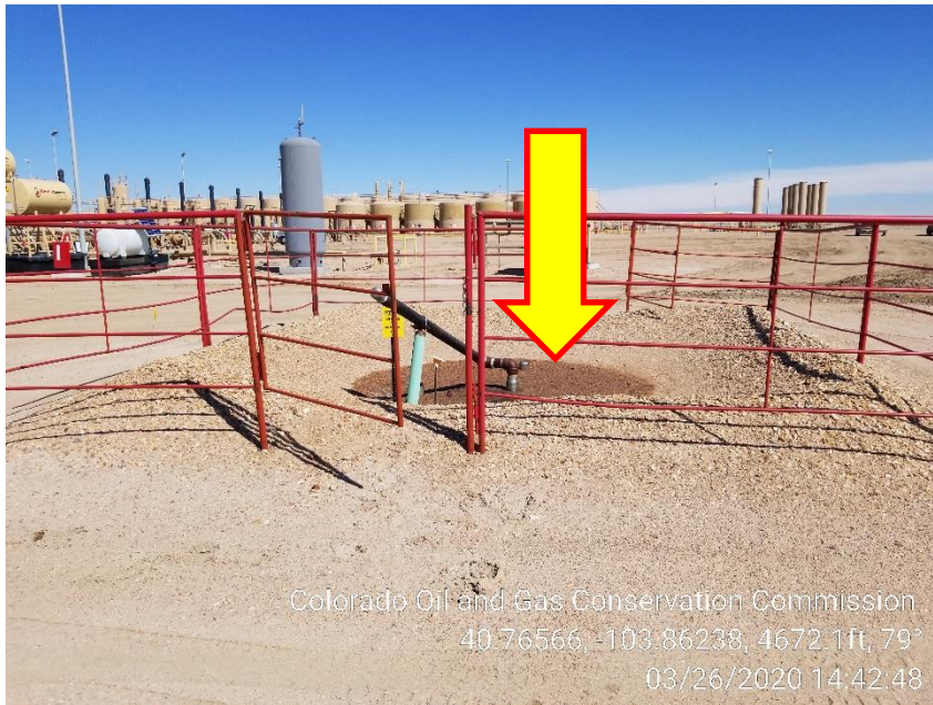
Photo 11 – Compressor Drain tank – missing Signage and Stained Soil
