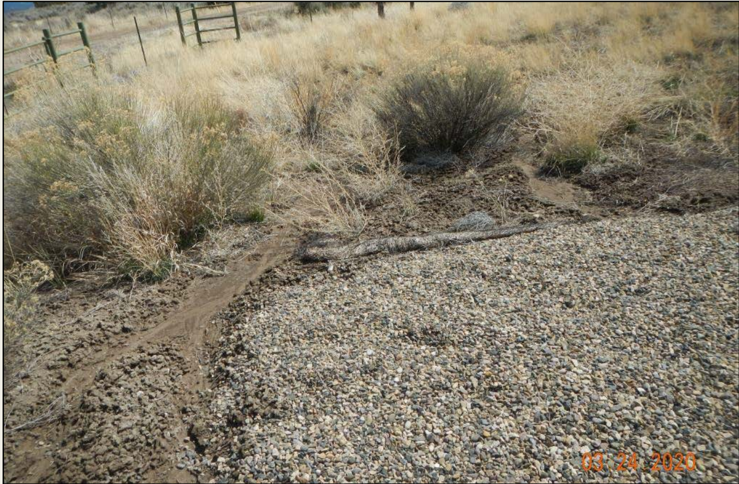
Photo 3. View of erosional channeling and failed wattle within the northeastern corner of the working area.
