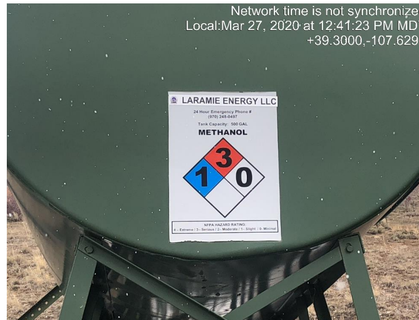
Photo #0854 1000 gallon methanol tank capacity not accurate.
