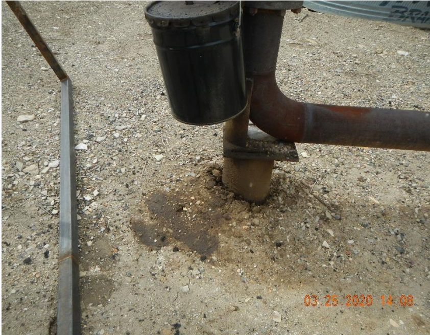
Stained soil at exhaust.
