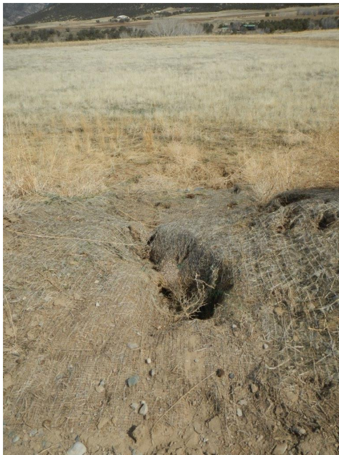
Photo#3: Stormwater issue at East side berm.
