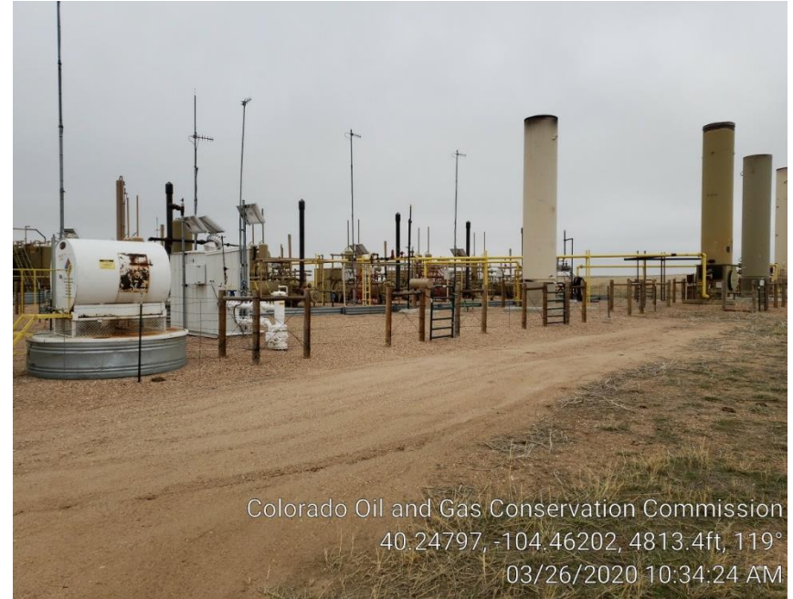
Photo #10 Separators, ECD's & Meter Run
