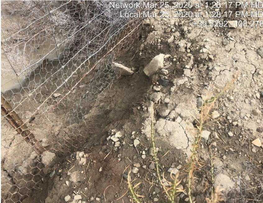
Photo #0830 Hole in wildlife protection device.
