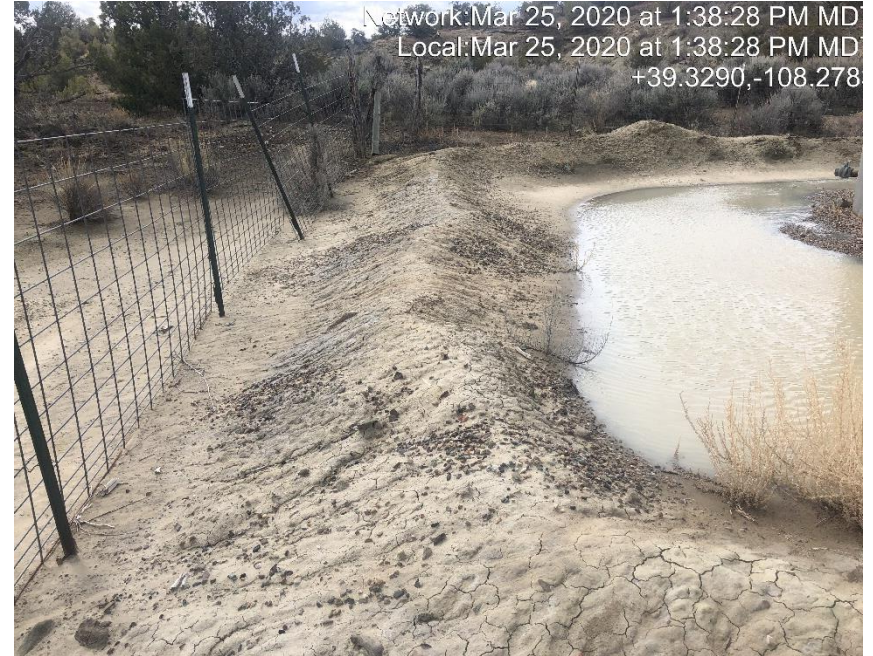
Photo #0834 Tank containment berm needs repaired.
