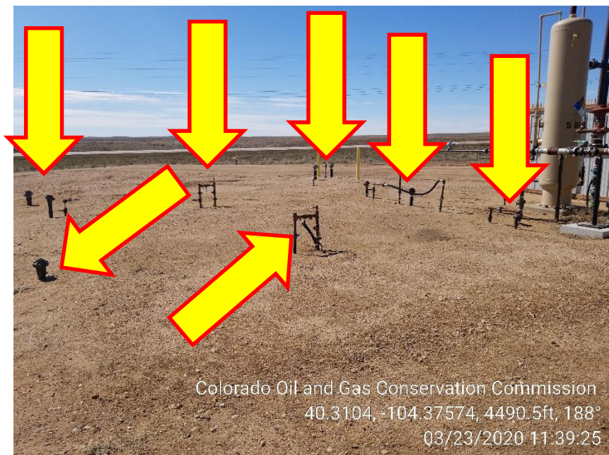
Photo 15 – Unmarked 1" Risers
