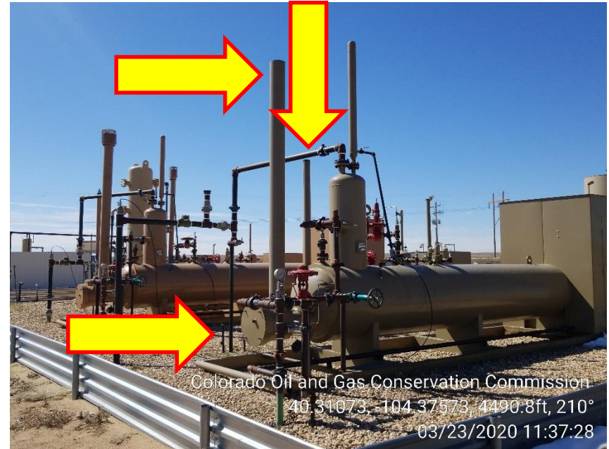
Photo 10 – North 2 Separators are missing Wildlife screens. Unmarked 1" Risers
