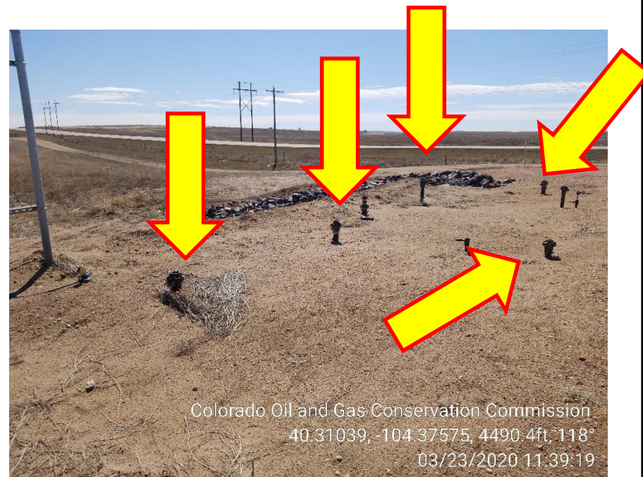
Photo 14 – Unmarked 1" and 2" Risers
