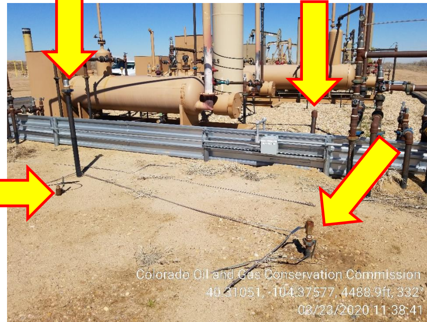
Photo 12 – Unmarked 1" and 2" Risers
