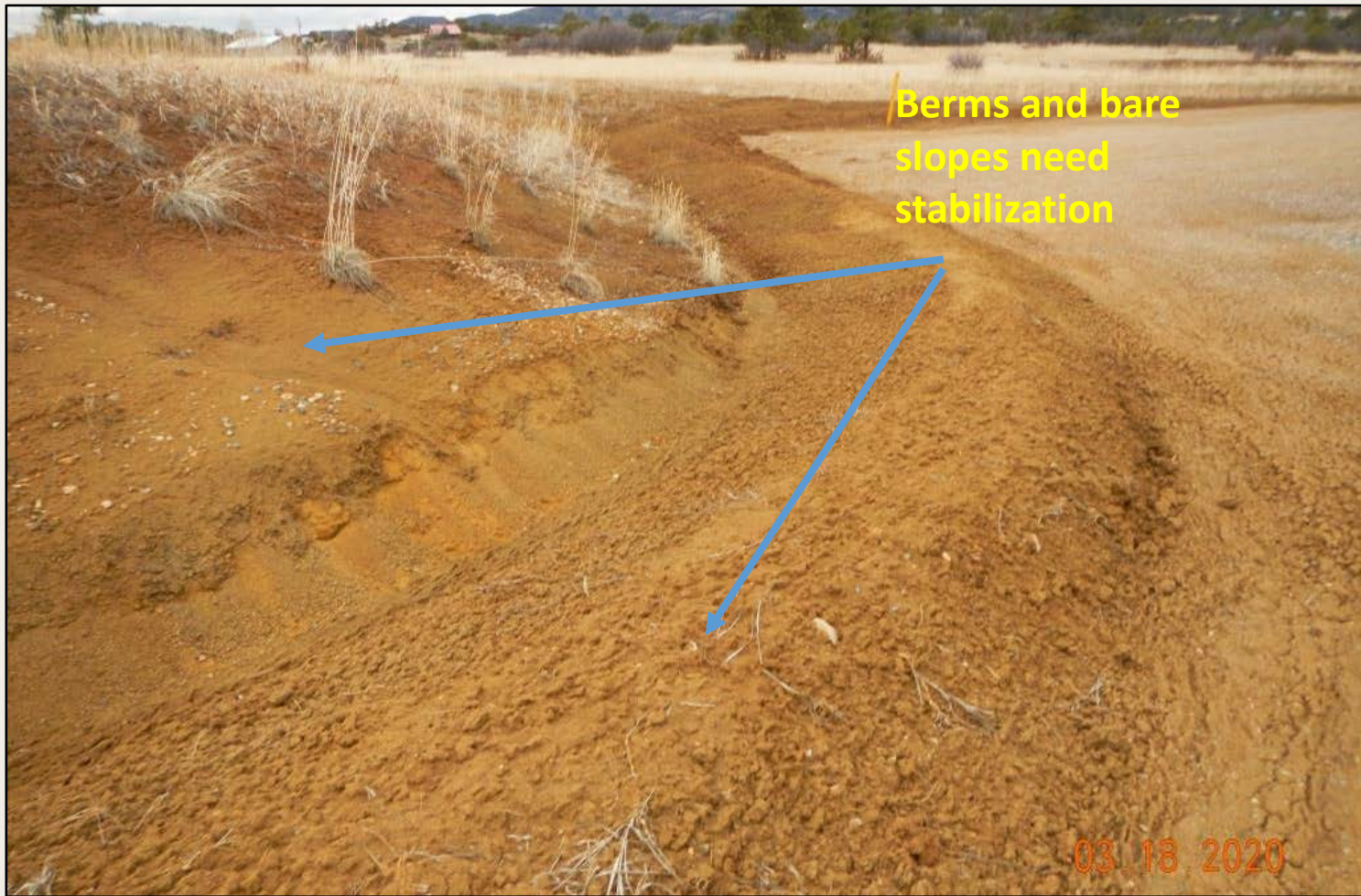
Photo 4. View of the southwestern edge of the well pad working area facing westward from the well pad entrance. Berms and eroding slopes need stabilization.
