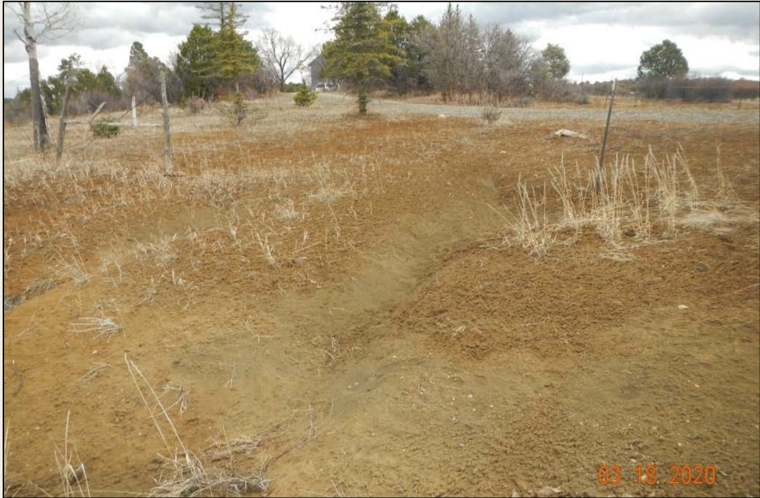
Photo 3. View of area near well pad entrance where stormwater run-on is eroding down-slope toward the access road. Stabilization measures are needed here.
