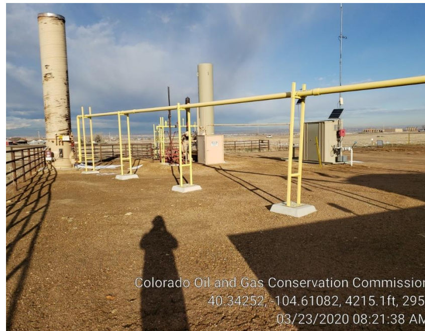
Photo #2 Separator, ECD's & Meter Run
