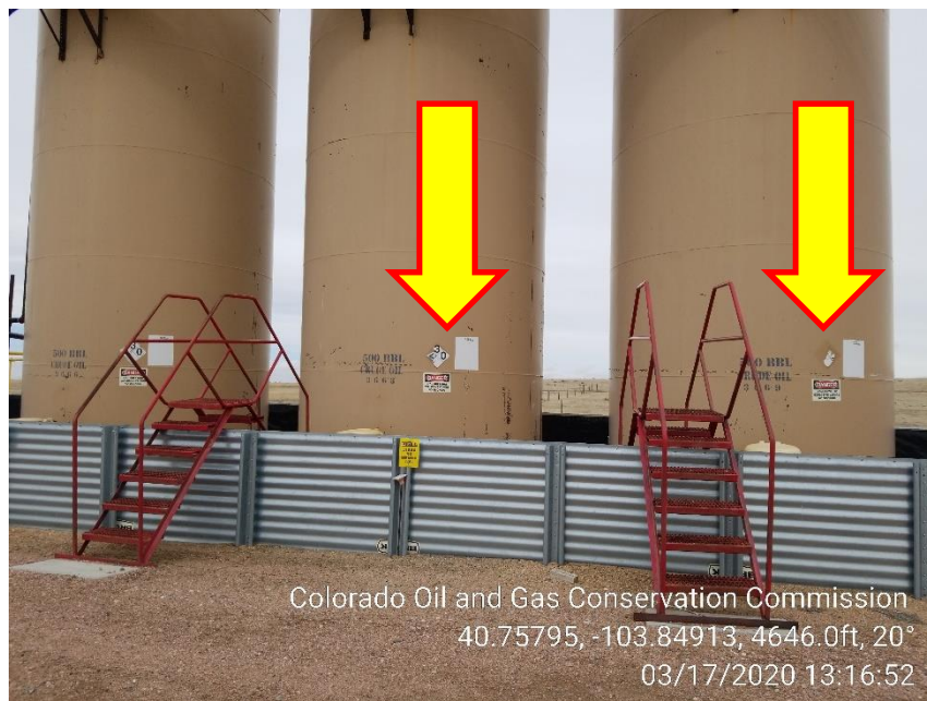
Photo 5 – Tank Labels Fading/Peeling
