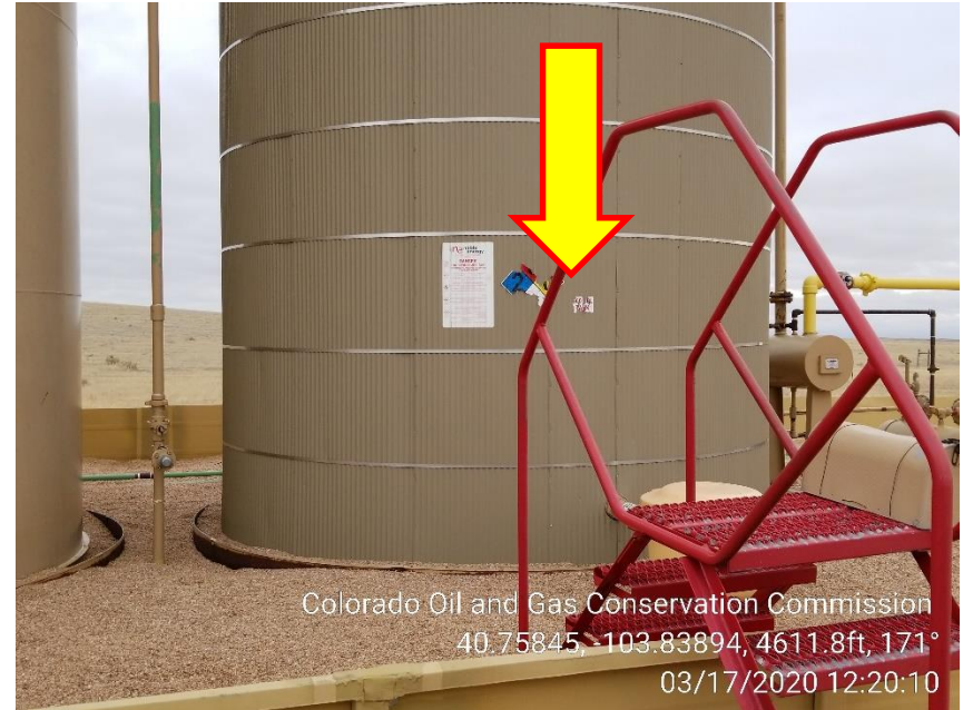
Photo 4 – Produced Water Tank – Missing Content. NFPA and Capacity labels are fading/peeling off.
