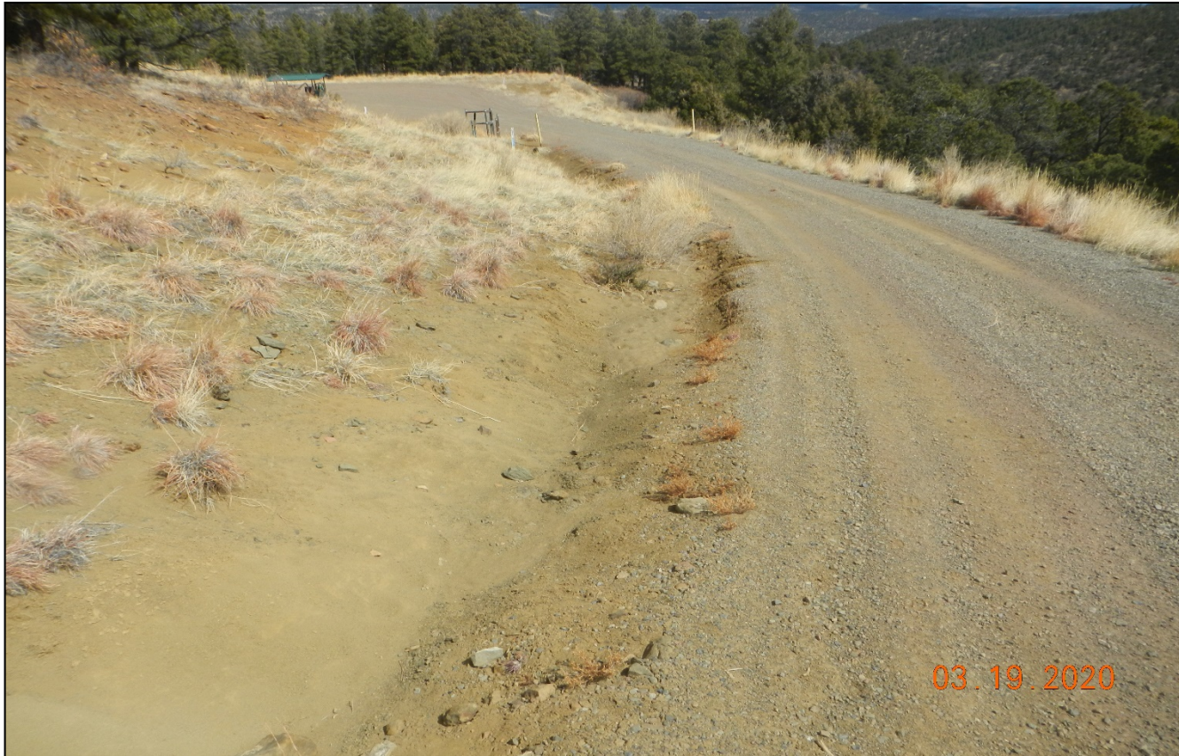
Photo 5. Erosion is occurring along the side of the road near the location.
