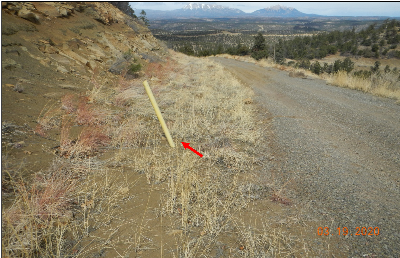
Photo 3. There are multiple culverts filled in with sediment along the access road.
