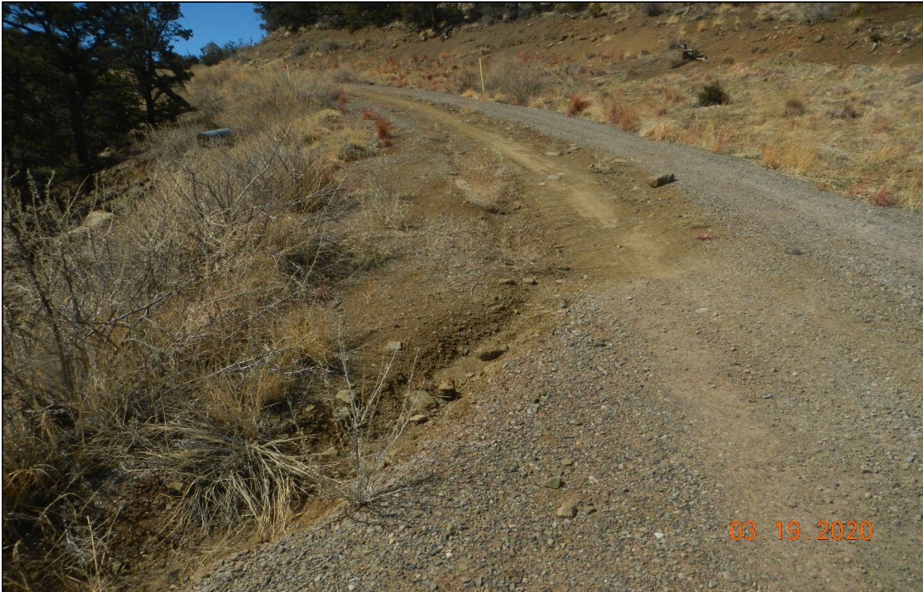
Photo 4. Facing back to the southwest along the access road. Stormwater is causing erosion down the road and is not properly diverted.
