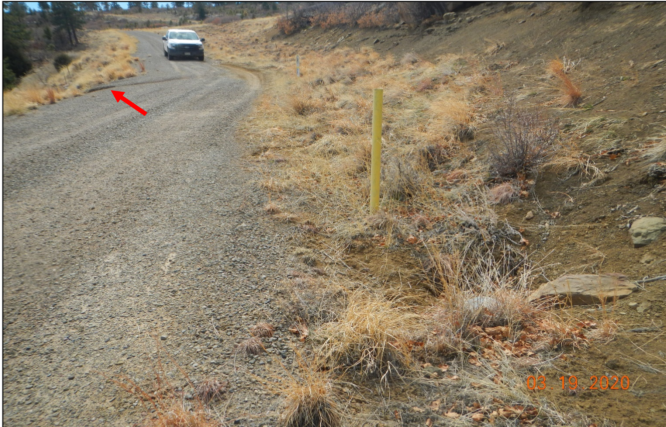
Photo 2. The culvert along the access road is filled in with sediment. Arrow points to erosion shown in previous photo. Stormwater needs to be diverted to the culvert.
