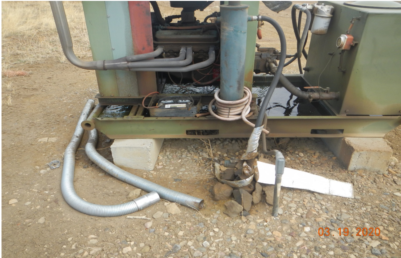
Photo 5. The is oily water in the engine skid.
