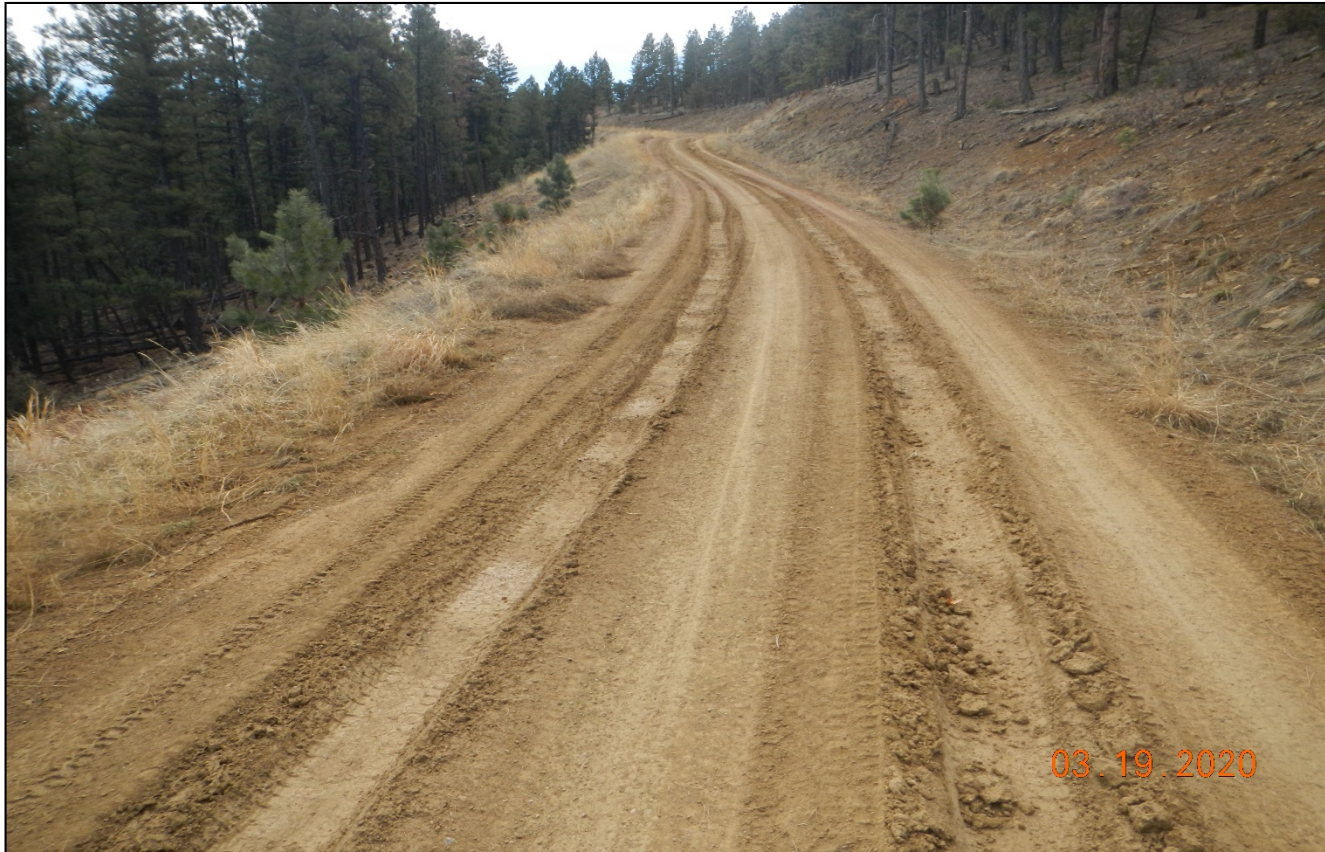
Photo 1. Facing southeast along the main lease road ascending the hill. There are vehicle ruts along the road. The road needs to be graded and maintained.
