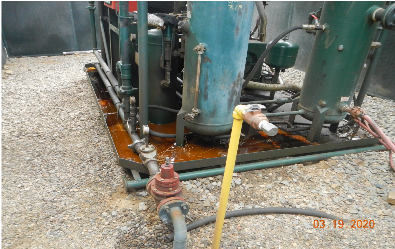
Photo 7. There is oily waste in the engine skid at compressor.
