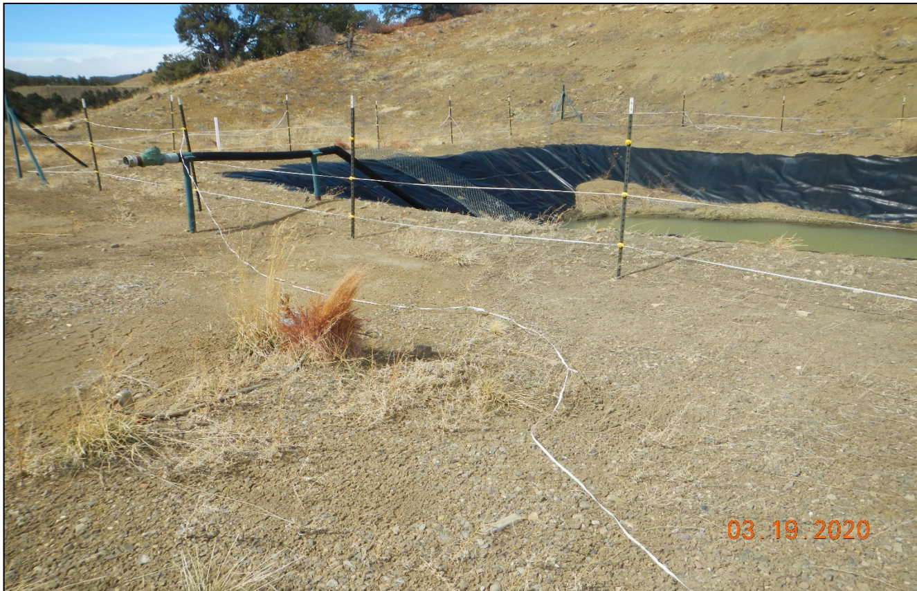
Photo 2. The electric fence around the pit is in disrepair and needs to be maintained.
