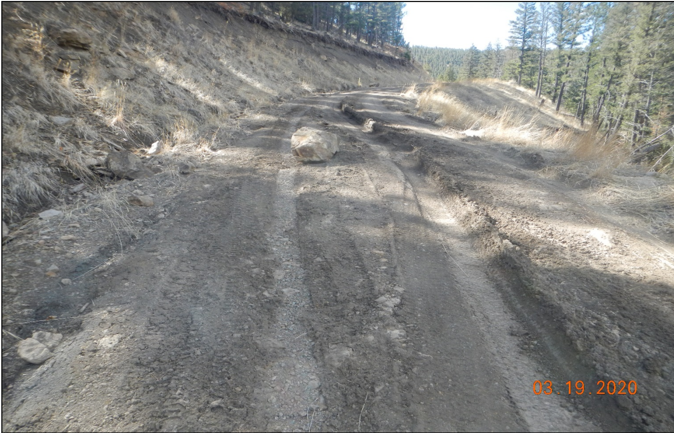
Photo 2. Facing west along the access road. There is a large rock in the road and deep vehicle ruts along the road.
