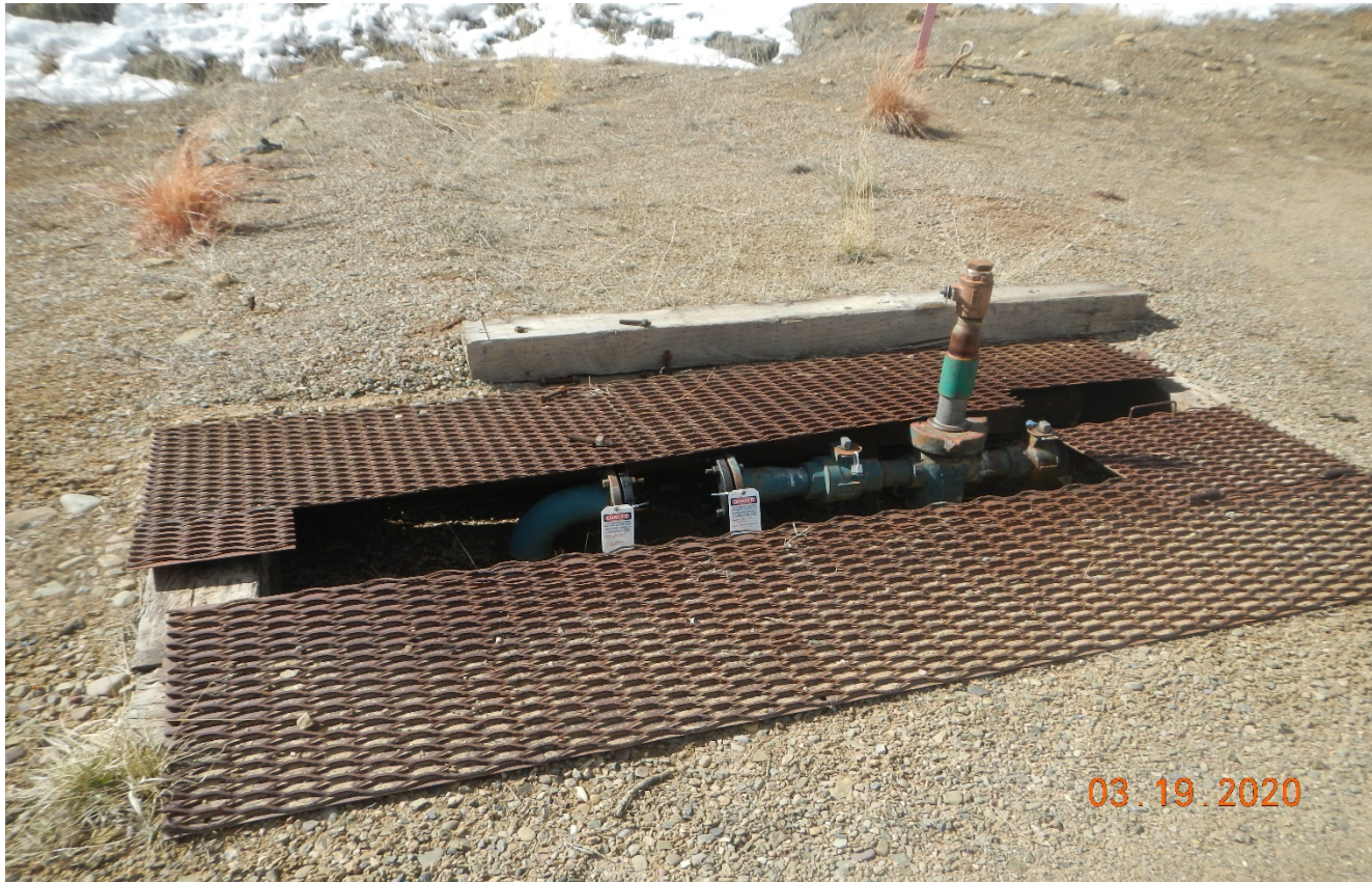
Photo 5. The pipe risers have been LO/TO.
