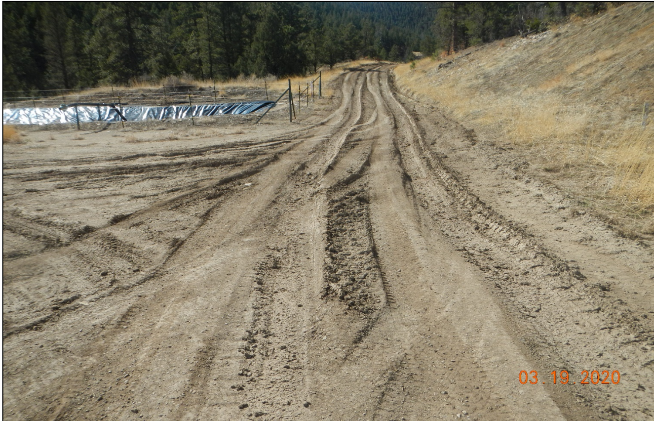
Photo 1. Facing southwest along the access road near the GE 31-04 site. There are vehicle ruts along the road. The road needs to be graded and maintained.
