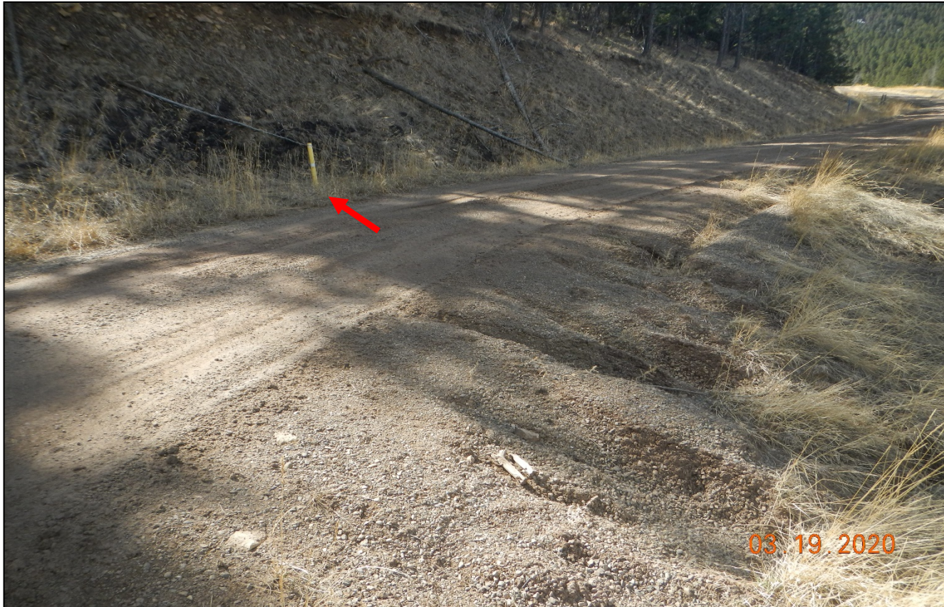
Photo 3. The culvert inlet shown at red arrow is filled in with sediment causing stormwater to flow across the road causing erosion.
