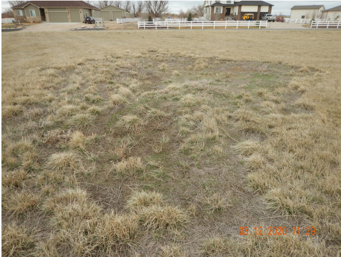
Photo 4. Photo taken from the plugged and abandoned well, facing Southwest. Photo illustrates the well location has not been properly recontoured due to subsidence.
