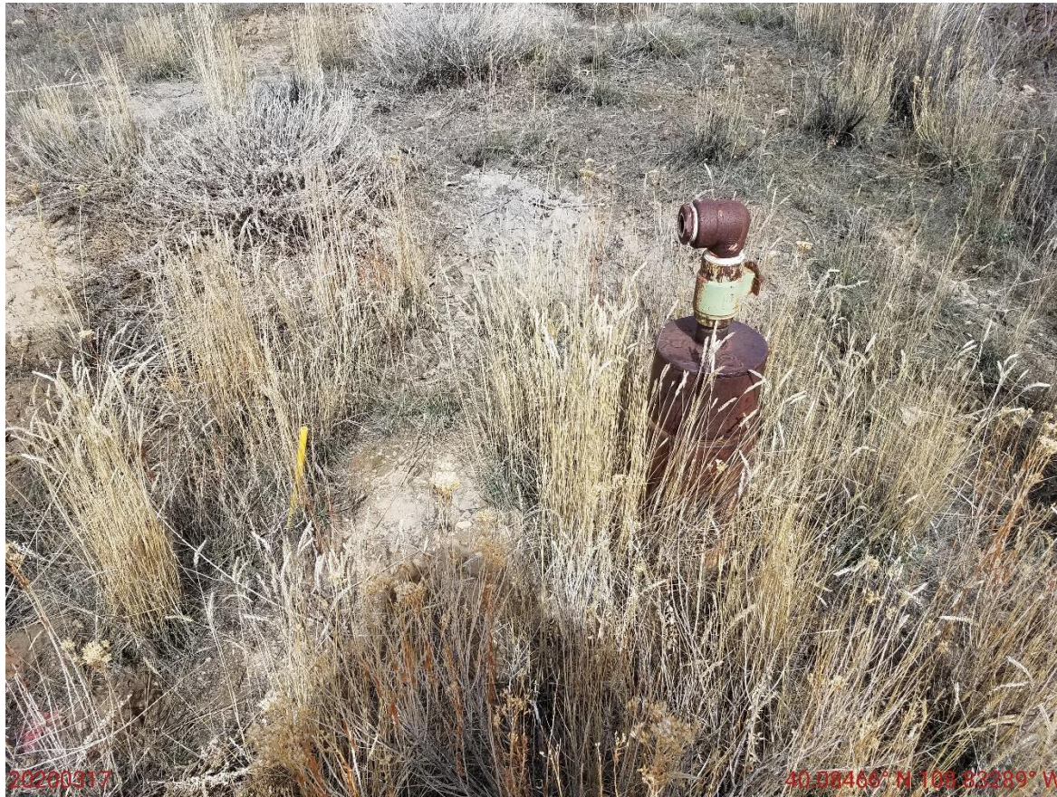
Photo 2: Photo shows well casing; Well does not appear to have been sufficiently plugged or cut/capped or in compliance with Rule 319.a.(5).
