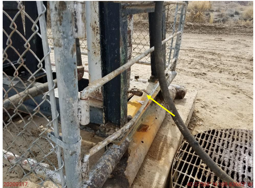
Photo 8: Photo taken from the well head. It was observed that gas appears to be venting from equipment attached to the bradenhead. Arrow shows open valve where gas appear to be venting from.
