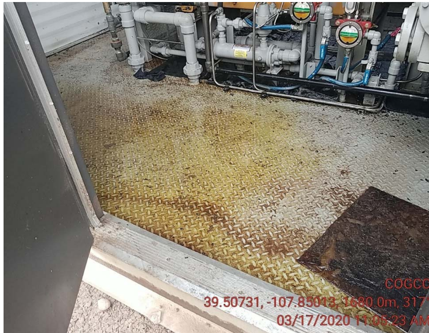
oil on the floor of compressor building
