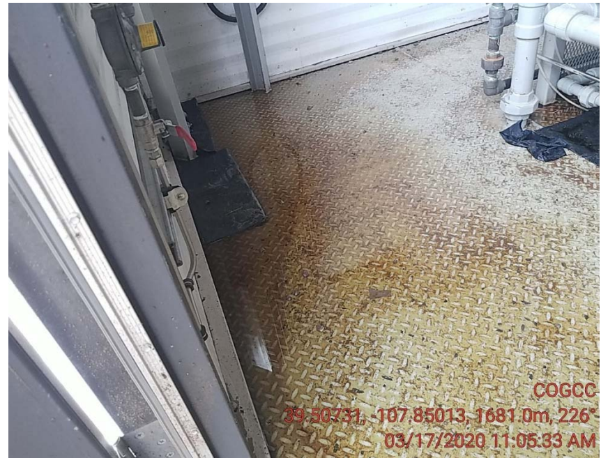
oil on the floor of compressor building
