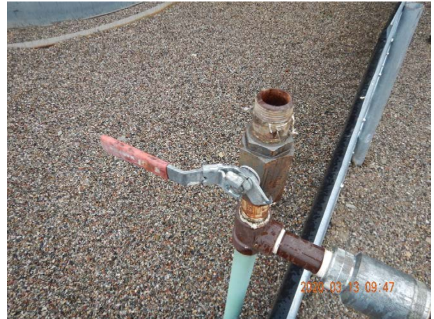
Photo #4 – Uncapped, unmarked flowline riser on south side of tank battery.
