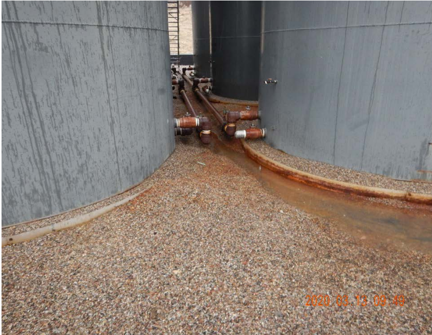
Photo #7 – Unidentified fluids inside of tank battery, view from south.
