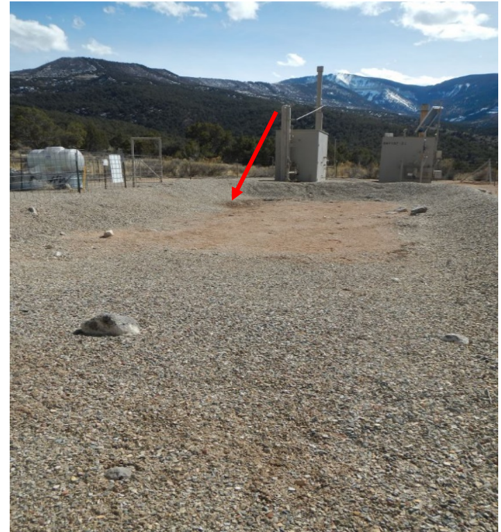
Photo#3: Hole developing in containment.
