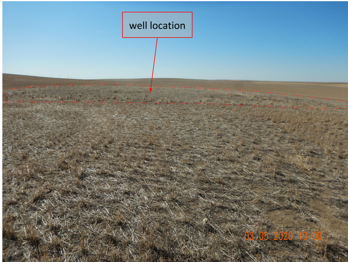
Photo 2. Photo taken from north of the well location, facing South. Photo illustrates Operator has not properly contoured the well location (within the red-dashed area) to match the surrounding landscape.
