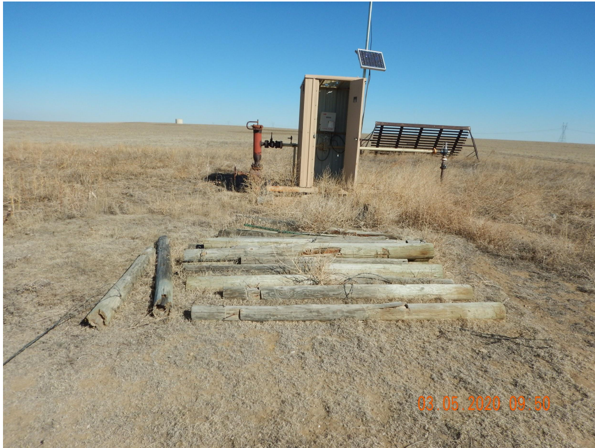
Photo 1. Photo taken from the southern tank battery location, facing North. Photo illustrates Operator has failed to remove equipment and debris from location and conduct reclamation of the location.
