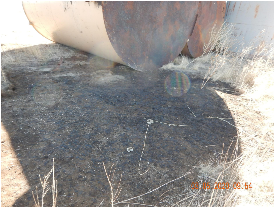
Photo 7. Photo taken from the tank battery location, facing East. Photo illustrates Operator has failed to clean up and remediate contaminated soils from a leaky tank.
