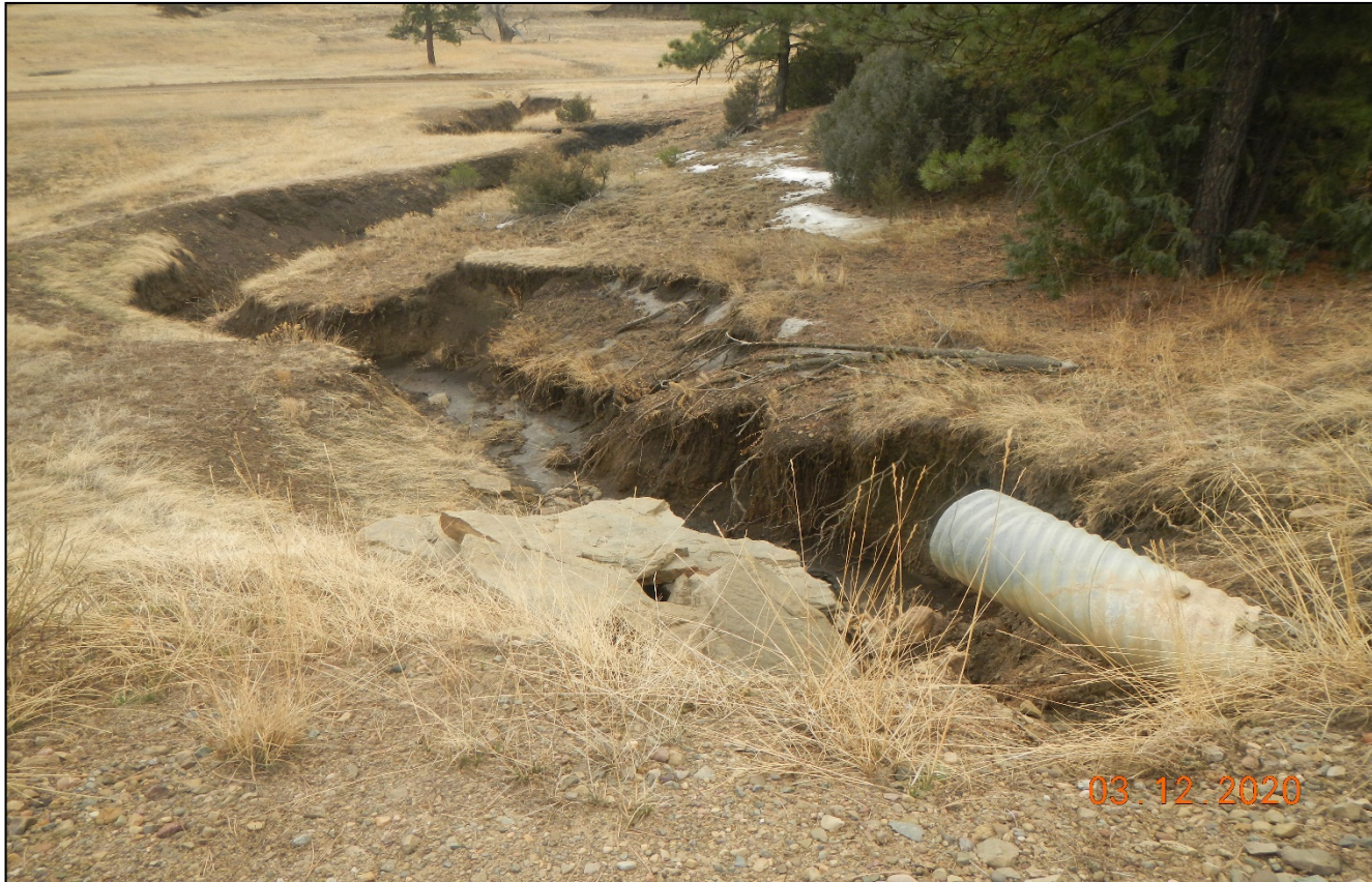
Photo 1. There is erosion occurring at this culvert outlet along the main road at Lat/Long:37.05979,-104.81561. No culvert outlet BMP to prevent erosion. Stormwater is being directed to this area from the road.
