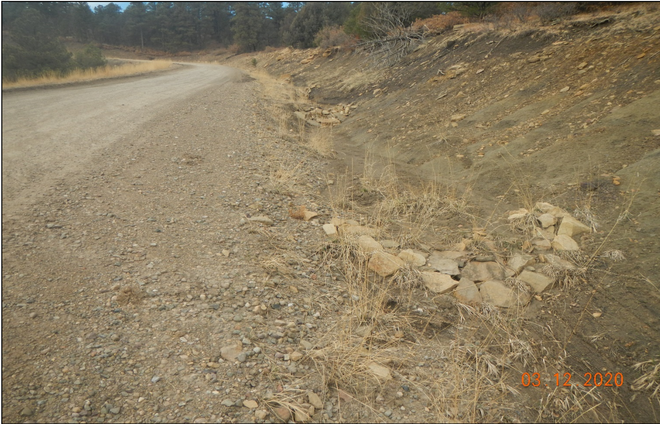
Photo 3. Erosion is occurring on the side of the road and rock check damns have filled up with sediment at Lat/Long:37.0586,-104.81750.
