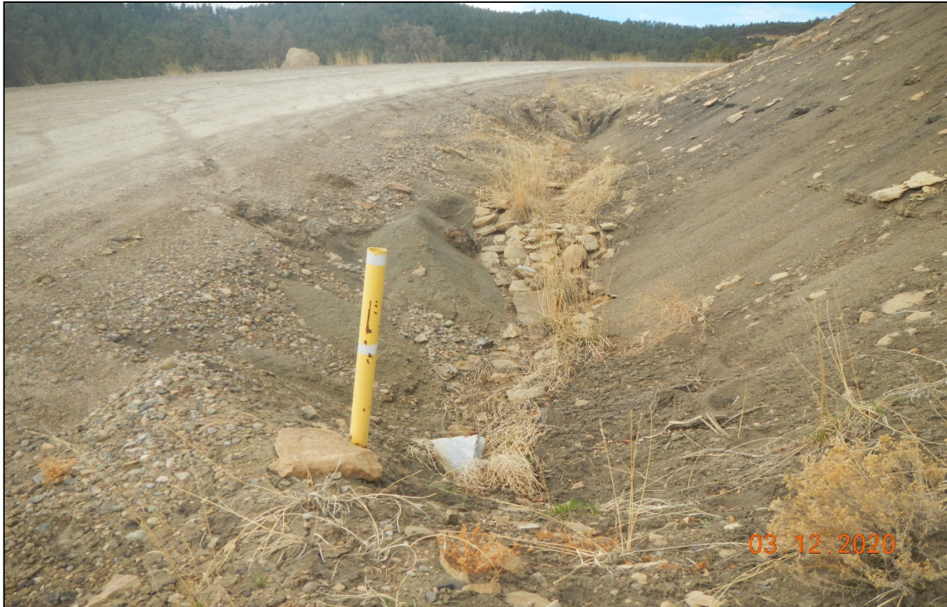
Photo 4. Erosion is occurring on the side of the road and this culvert has filled in with sediment at Lat/Long:37.0586,-104.81750.
