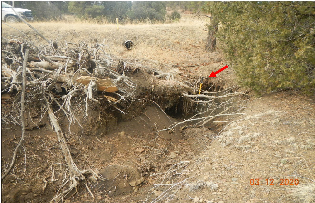
Photo 2. Further up the road there is erosion occurring from the culvert outlet along the main road at Lat/Long:37.05963,-104.81659. No culvert outlet BMP to prevent erosion. Red arrow points to 4.5 foot shovel placed in erosion gully.
