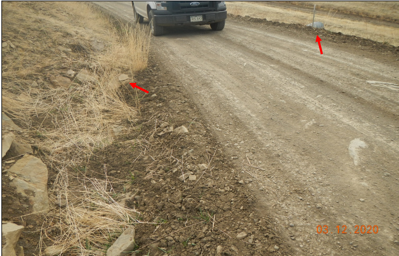
Photo 1. The culvert along the access road to the location has filled in with sediment. Arrow points to outlet and inlet.
