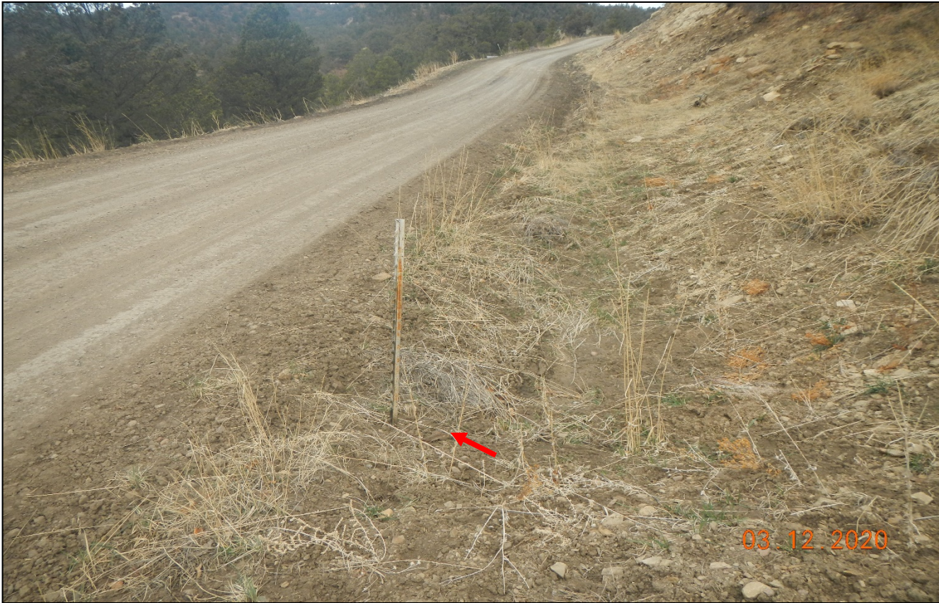
Photo 2. The culvert along the access road to the location has filled in with sediment. Arrow points to culvert inlet.
