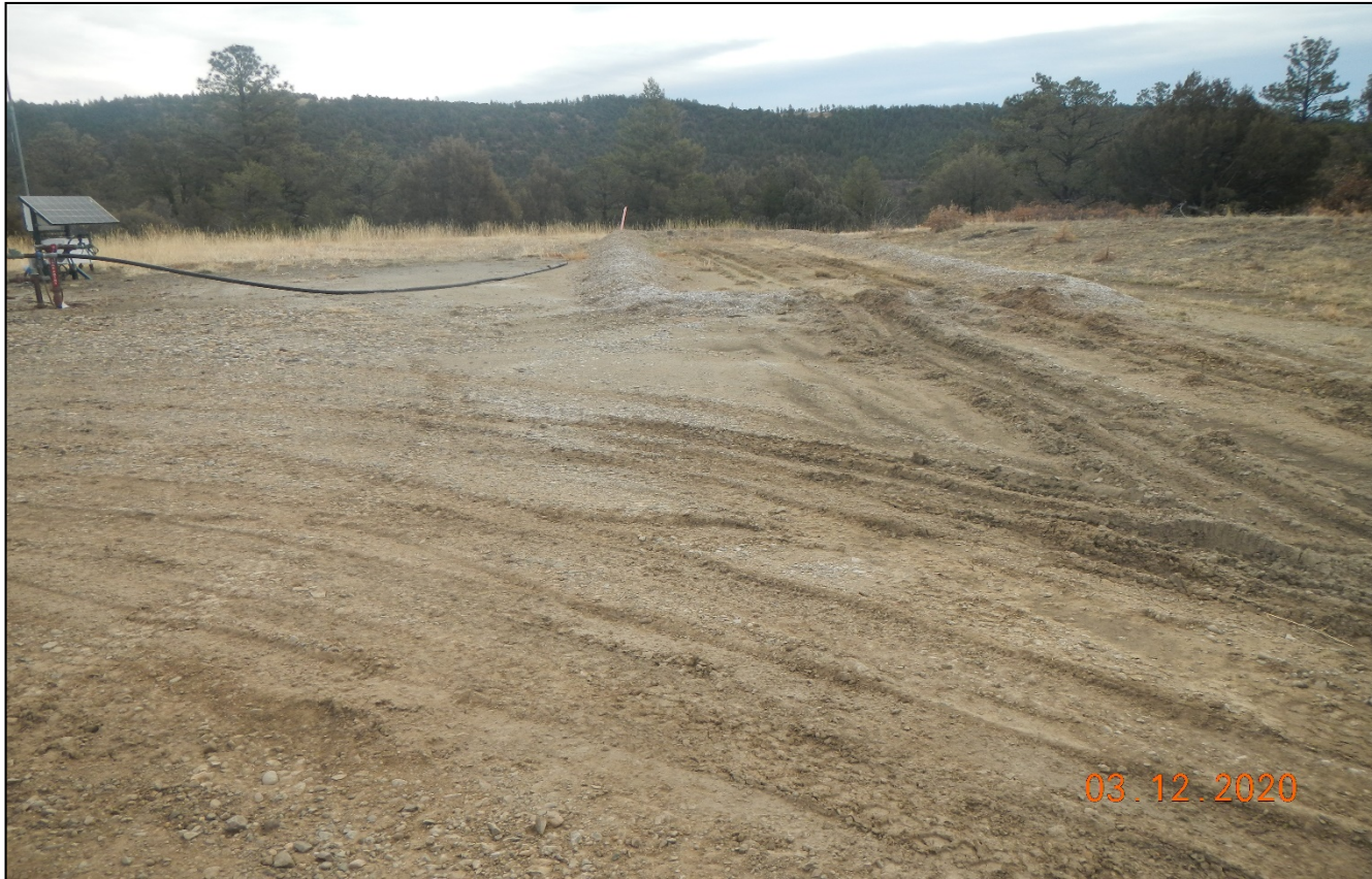
Photo 3. There is a berm that remains where water tank was located. This will need to be leveled and reclaimed in no longer in use.
