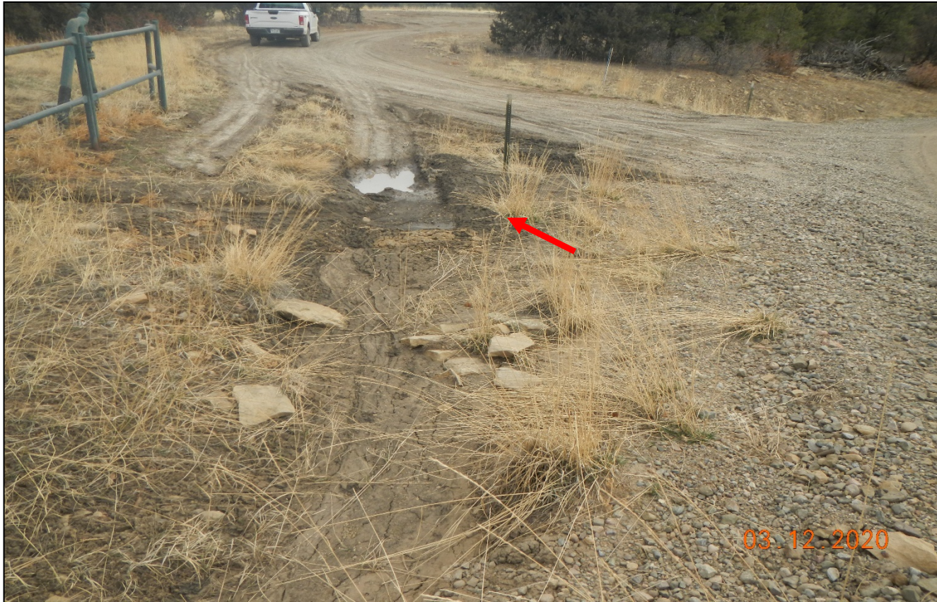
Photo 1. The culvert at the beginning of the access road has filled in with sediment. Arrow points to culvert inlet.
