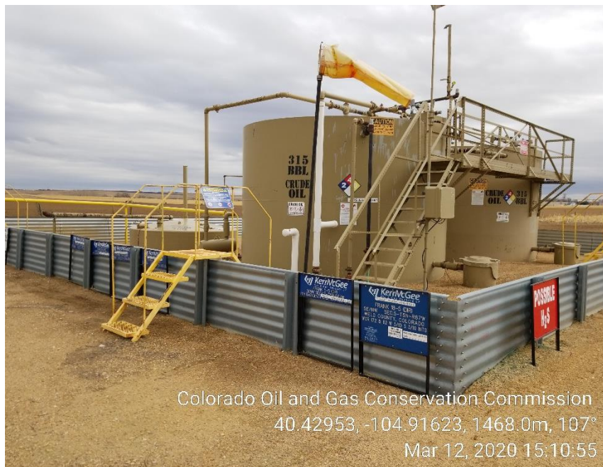
Photo 11: Tank Battery
