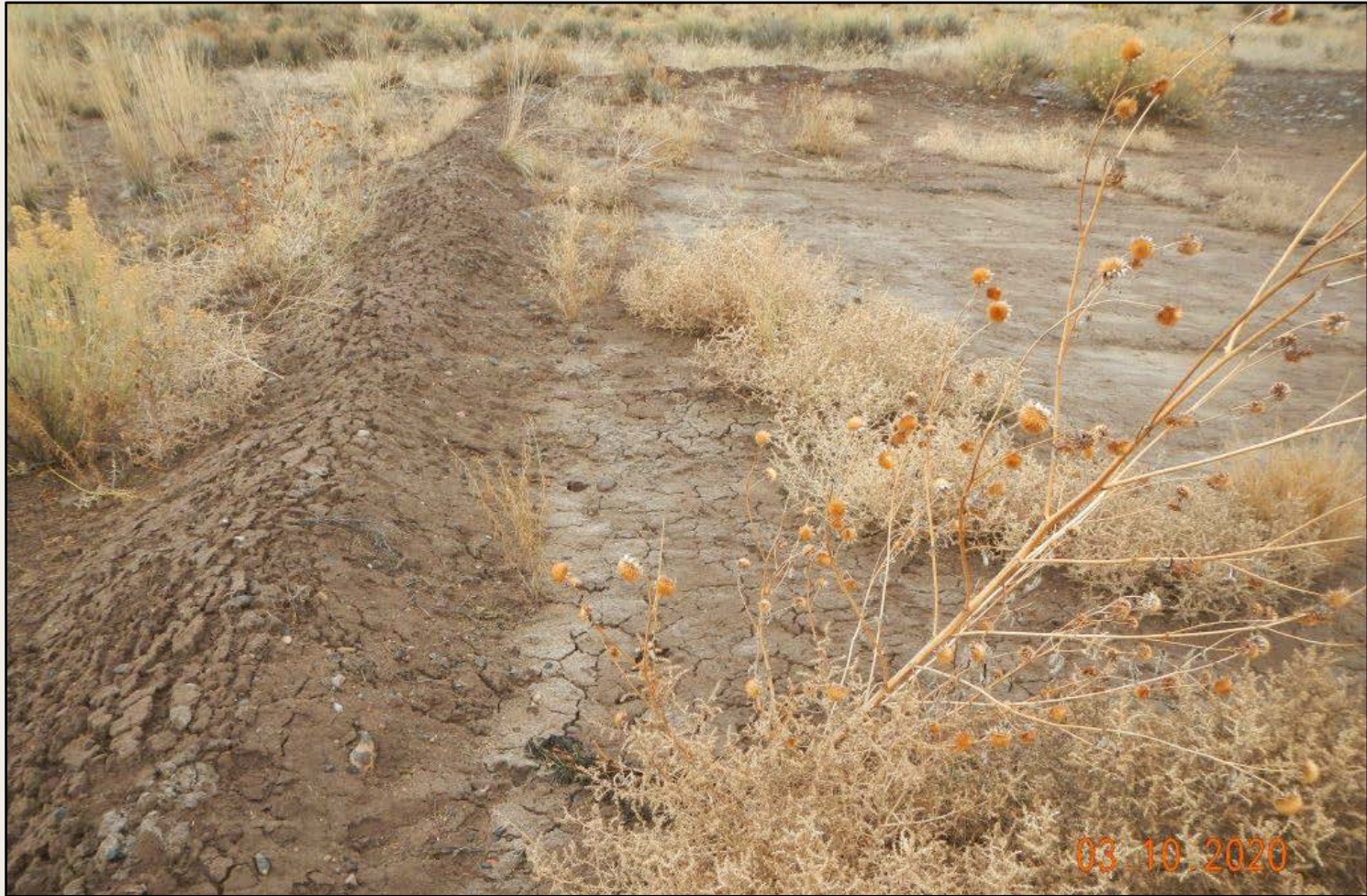
Photo 5. View of unconsolidated berm and bare soils within the southwestern project area, needing stabilization.
