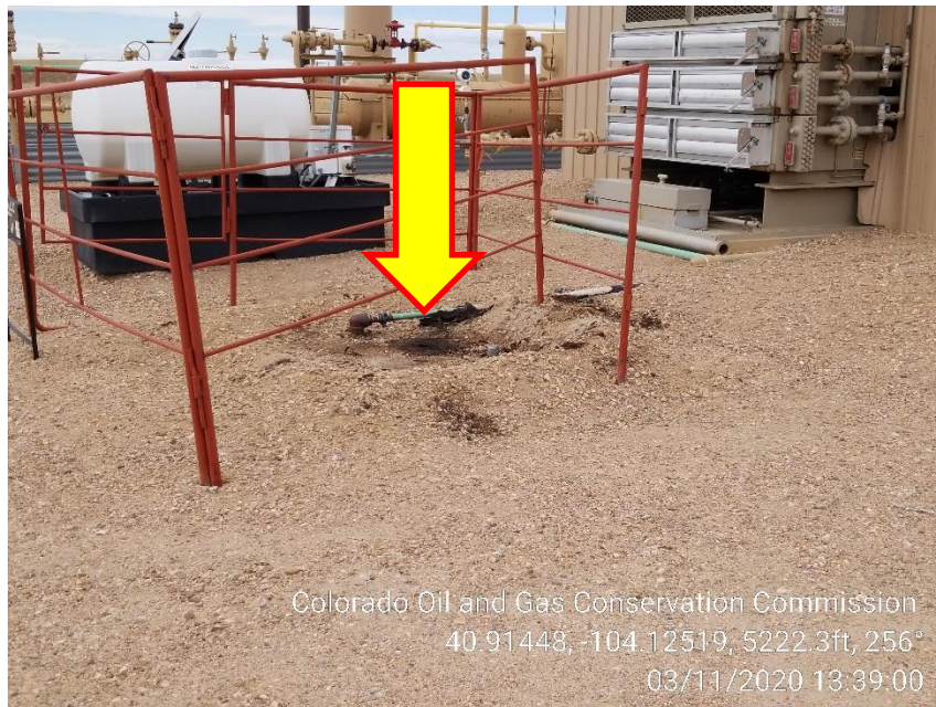
Photo 3 – Stained Soil at Compressor drain vault
