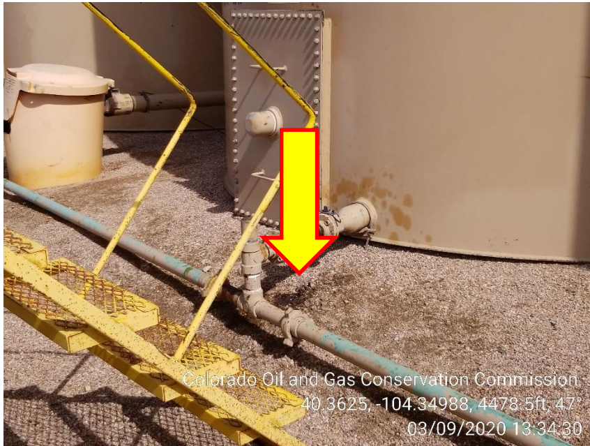
Photo 7— Stained Soil at drain valve
