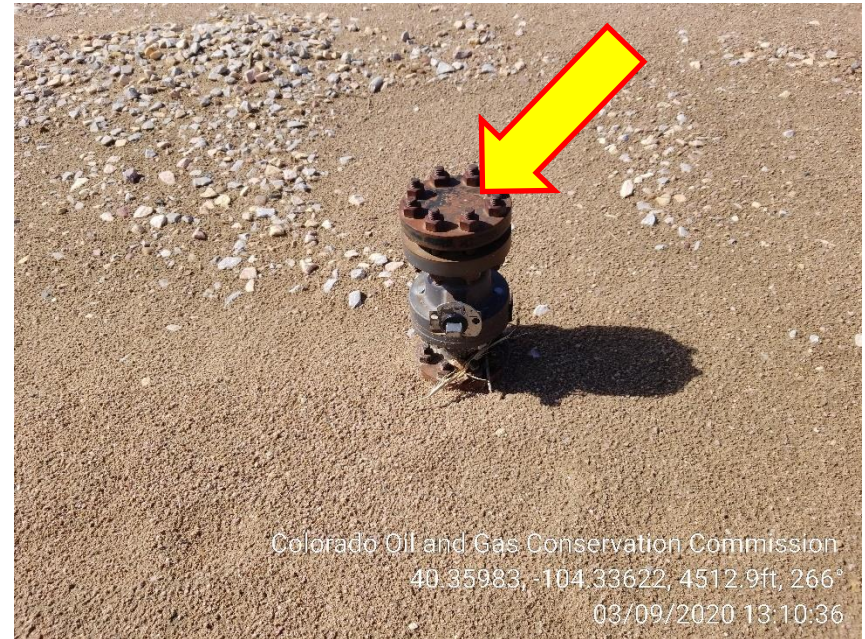
Photo 6 – Unmarked Riser
