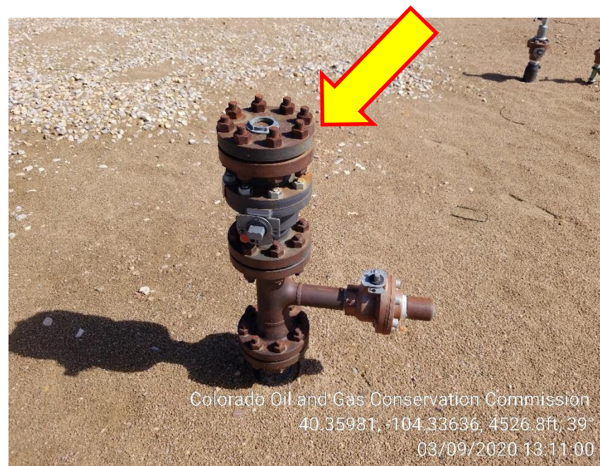
Photo 8 – Unmarked Riser
