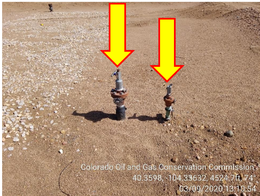
Photo 7 – Unmarked Risers
