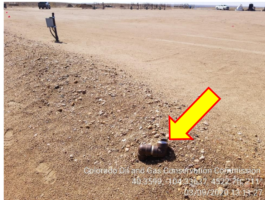
Photo 10 – Unmarked Riser
