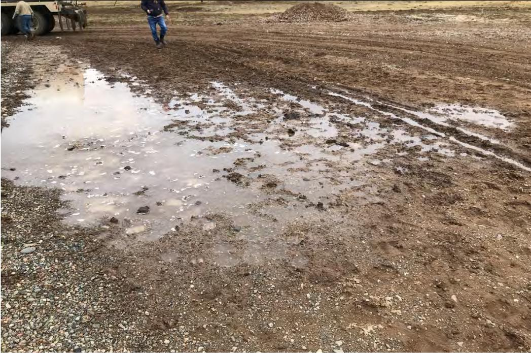
11/13/2019: Looking Southeast – Water truck recovering released water near terminus. Channels were trenched to flow as much water as possible to this point.
