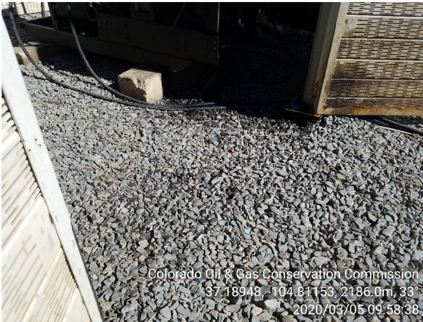
PHOTO 7: IMPACTED SOIL/GRAVEL NEAR PRIME MOVER ENGINE SKID. Conduct maintenance on equipment (ie REPAIR LEAKS ON ALL EQUIPMENT), cleanup stained material and review self inspection processes. CA DATE 4-5-20
