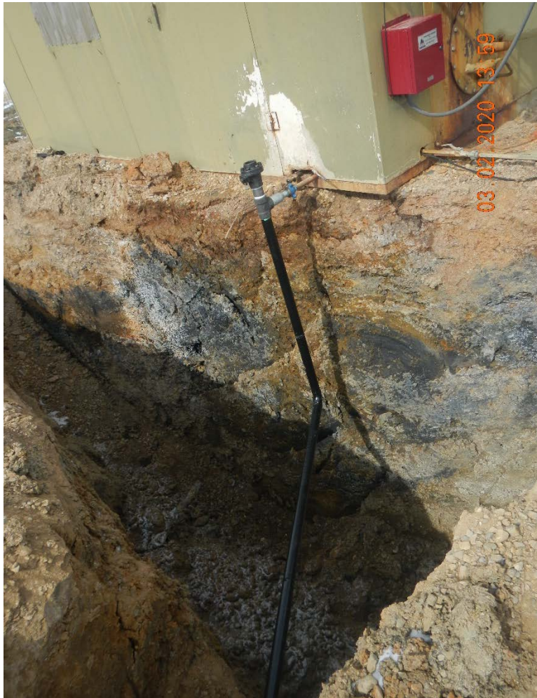
Photo #8 visually impacted soil below separator.
