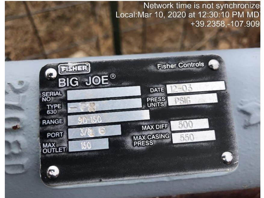
Photo #0742 Pressure plate of Big Joe regulator.
