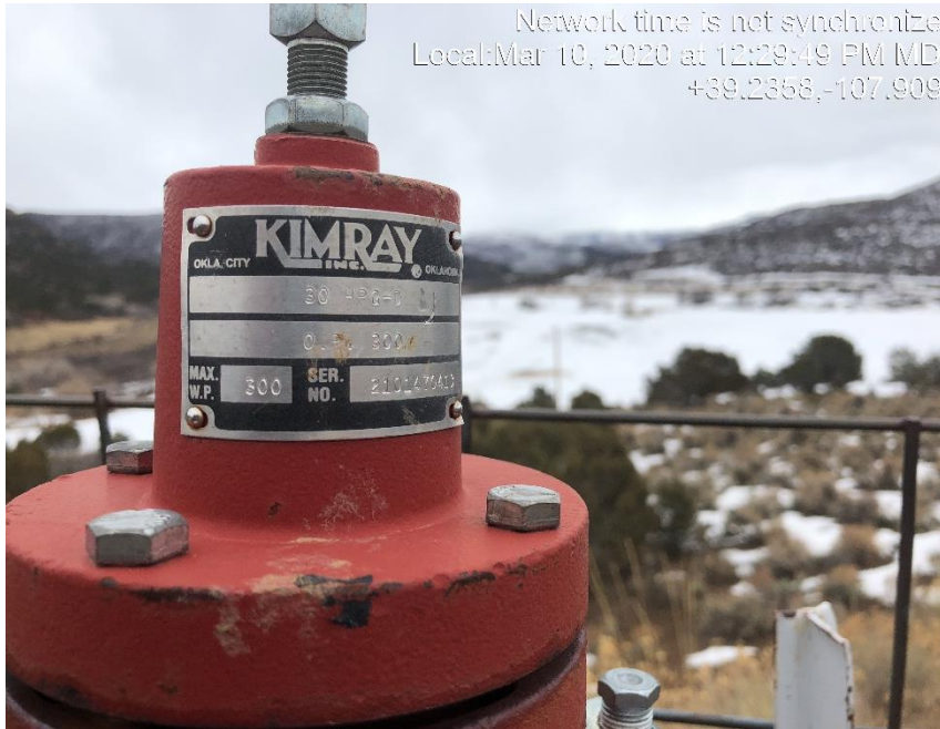
Photo #0740 Pressure plate of 1" Kimray regulator.
