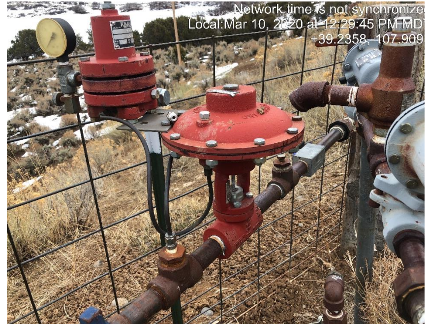
Photo #0739 Three in line regulators.
