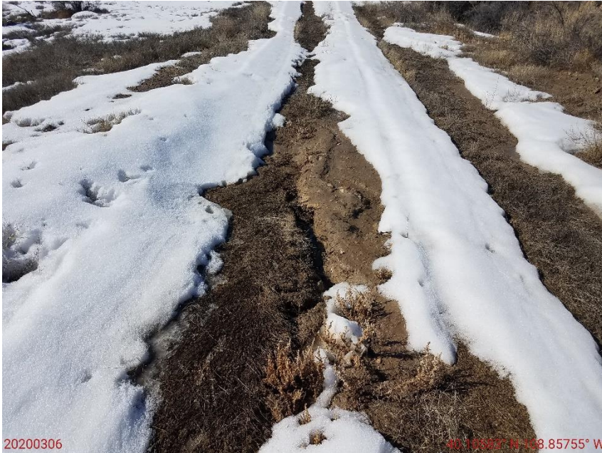
Photo 5: Photo shows erosion degradation on access road.
