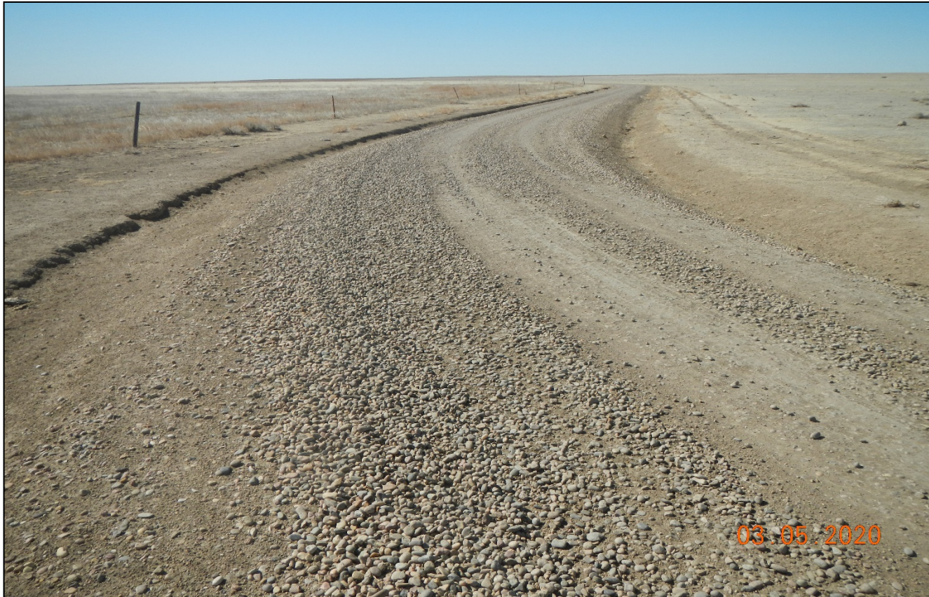
Photo 2. Facing southwest along the road. The road has been built up and graveled.
