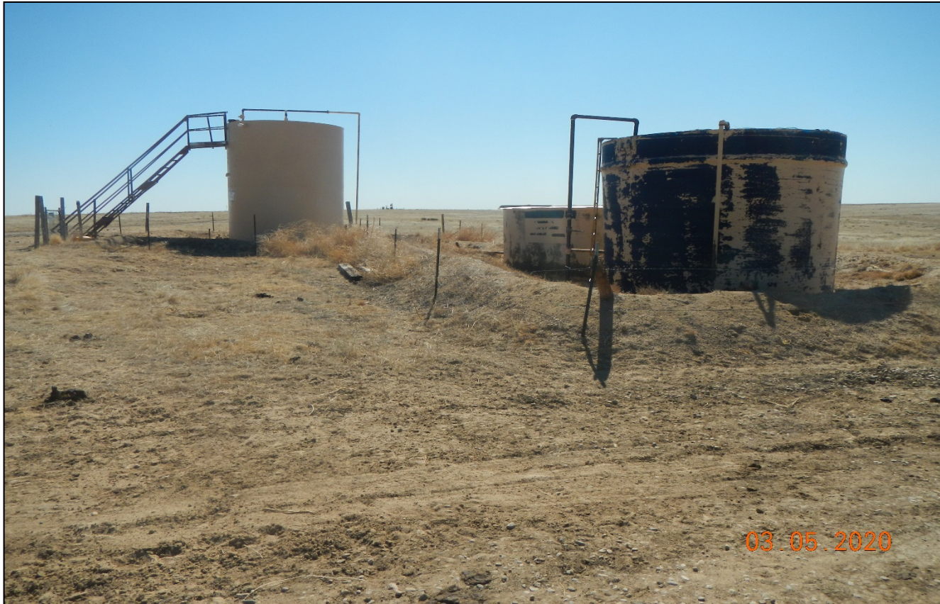
Photo 8. Facing toward the tank battery. Berms are maintained around tanks.
