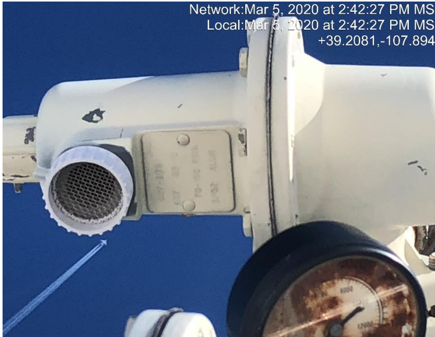
Photo #0710 Pressure plate of primary regulator.
