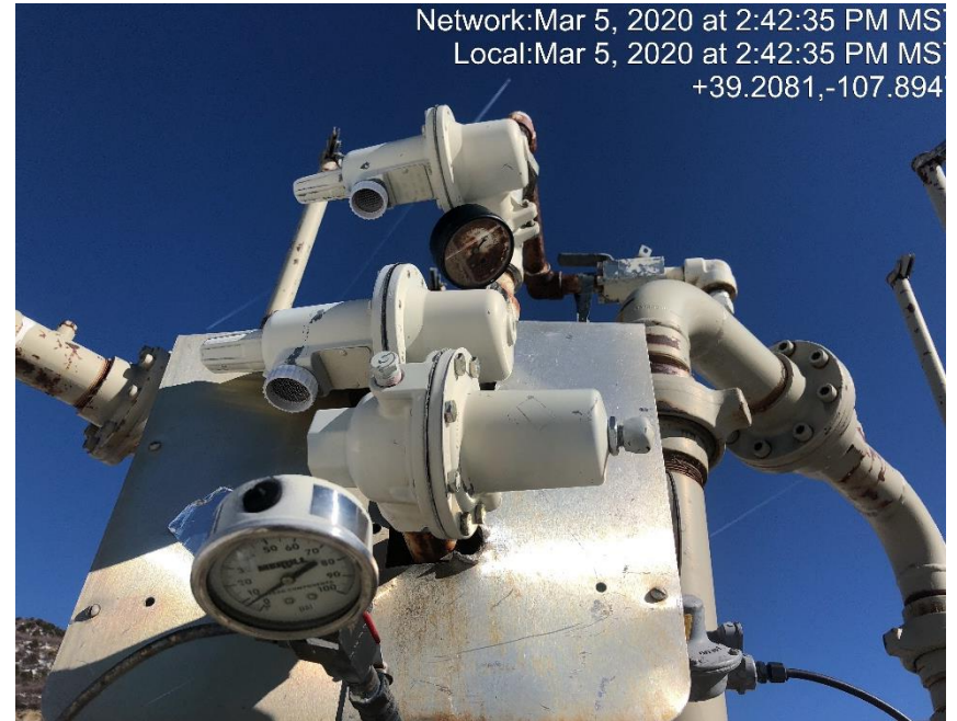
Photo #0711 In line Fisher regulators.
