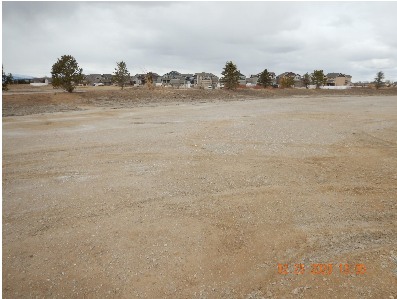
Photo 1. Photo taken from the well and tank battery location, facing Northwest. Photo illustrates Operator has removed all the major equipment but has not conducted surface reclamation (i.e., remove gravel, contour, ect...).
