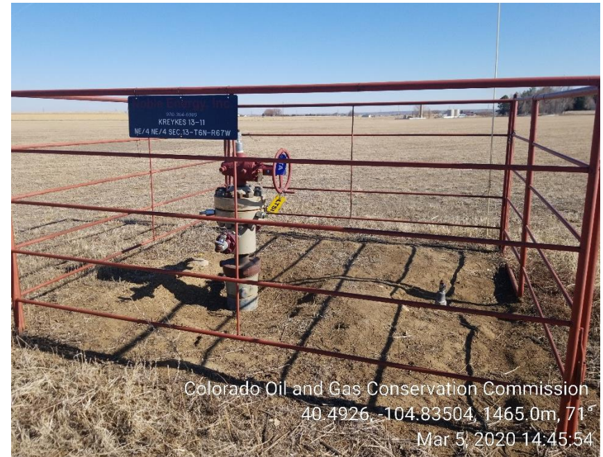
Photo 2: Wellhead; equipment removed
