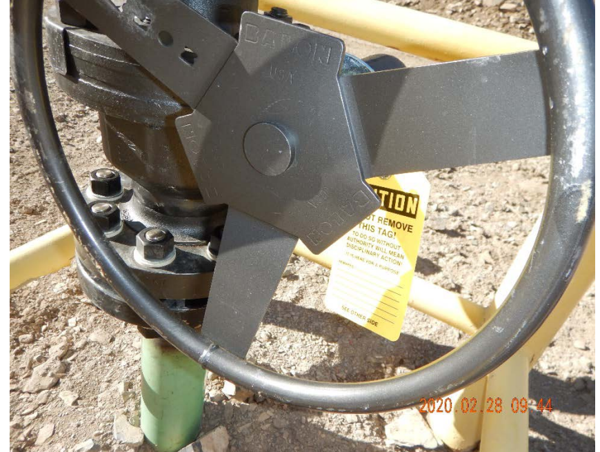
Photo #4 – Flowline on west end of pad was tagged out on inspection date.
