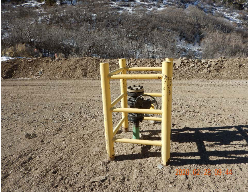
Photo #3 – Capped 4" flowline riser on west end of pad.
