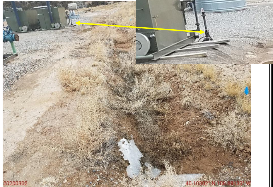
Photo 36: Continued from photo 35. Photo also shows riser identified in FIR 698100016 remaining on the Location; Corrective actions required Operator to remove riser.
