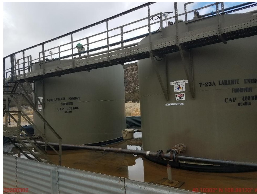
Photo 50: Photo shows the two (2) 400 BBL crude oil ASTs.
