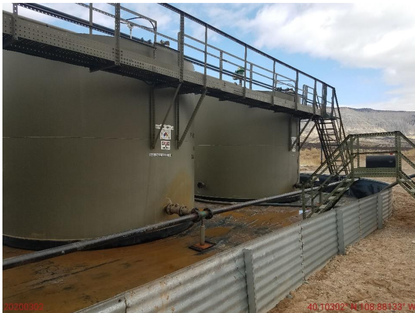
Photo 51: Photo shows the two (2) 400 BBL produced water ASTs.
