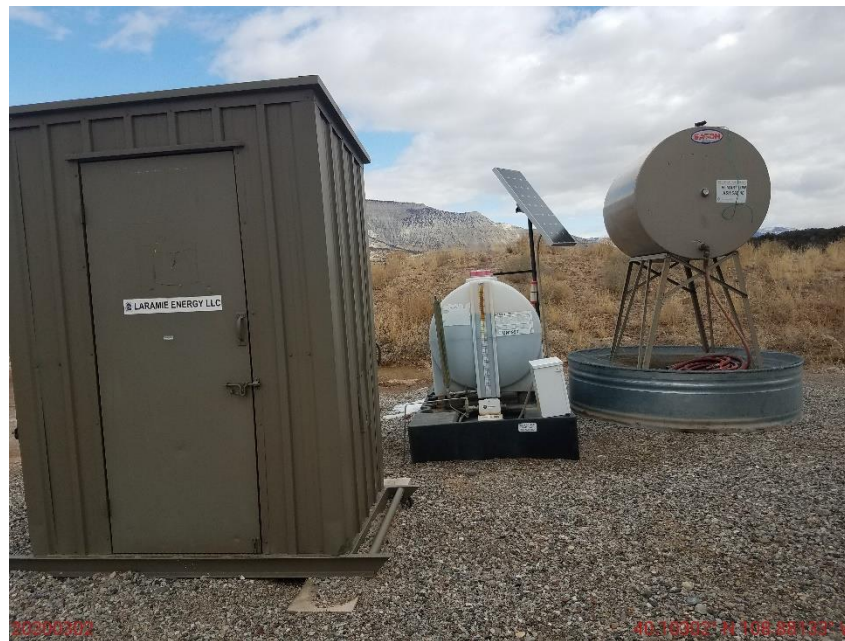
Photo 54: Photo of metershed, methanol tank and SAE 40 tank
